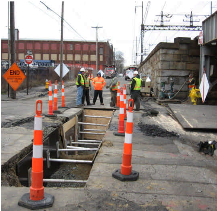
Both photos show trenching activities on Railroad Ave. at its intersection of Myrtle Ave. On the left, dewatering and filtering equipment is on-site in preparation for intercepting groundwater in the trench.
