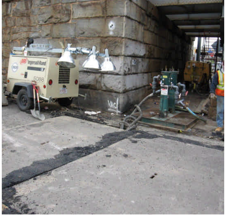
Both photos show trenching activities on Railroad Ave. at its intersection of Myrtle Ave. On the left, dewatering and filtering equipment is on-site in preparation for intercepting groundwater in the trench.
