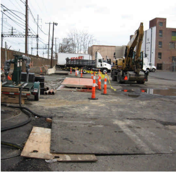
Left: Photo of trenching activities along Railroad Ave. at its intersection with Howard Ave. The sediment on the pavement adjacent to the filter equipment should be swept up and disposed of. Right: Oil spill on the pavement noted next to generator that should be cleaned as feasible.
