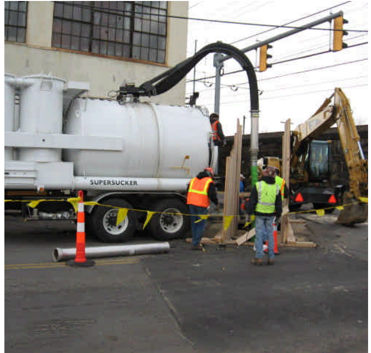
Both photos taken of trenching activities at the intersection of Railroad Ave. and Howard Ave. Left: Trenching activities in the adjacent parking area. Run-off was not noticeably turbid and was contained to the site. Right: Crews were using a vac truck to remove soil from around the existing utilities in the trench.
