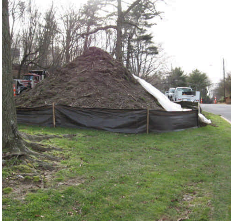
Both photos show trenching activities in the shoulder of Pequot Ave. near its intersection with Rt. 1. Left: Trench is being backfilled; erosion controls should be re-established at the close of each workday. Right: Soil stockpile associated with trenching activities. The pile remained stable and contained after a 1" rain event. Any sections of erosion controls in disrepair should be re-established.
