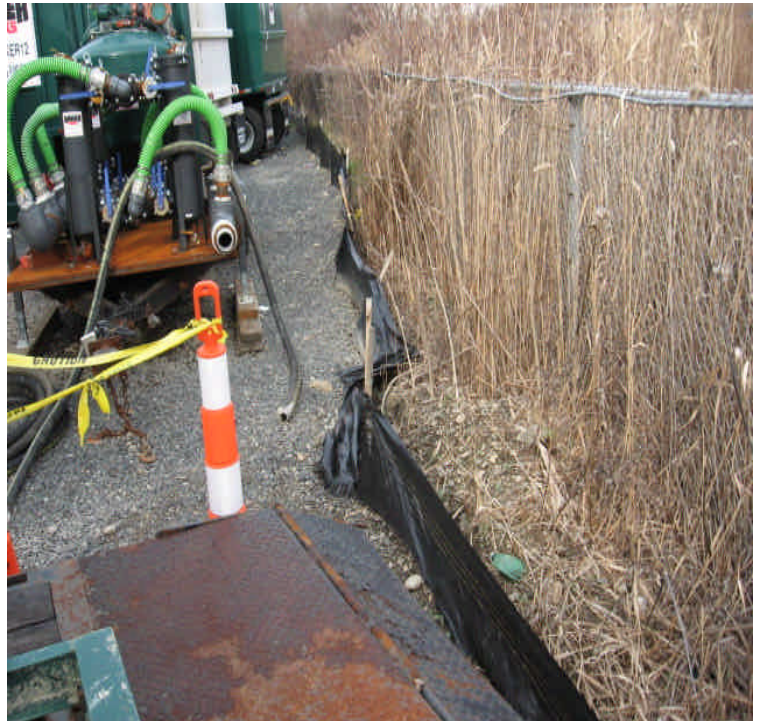
A small section of silt fence remains down near the entrance to the yard. The other side was repaired but controls here need maintenance.
