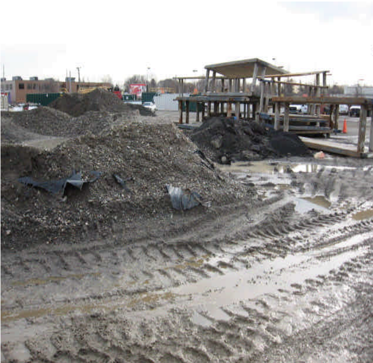
Concrete washout is not fully contained to the basin. It is recommended that improvements be made to contain all washout.
