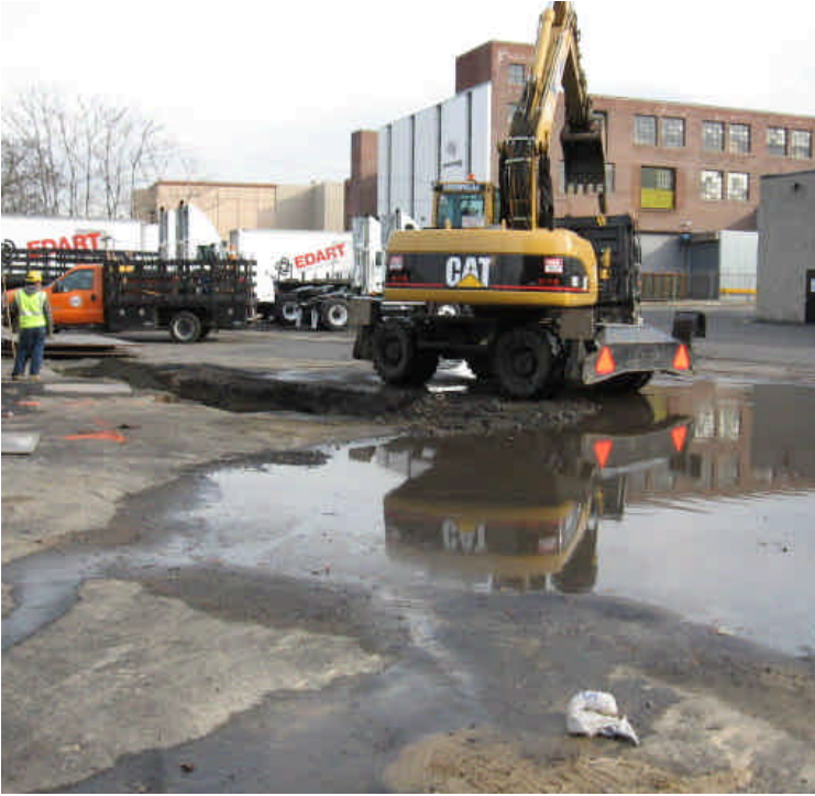
Both photos taken of trenching activities at the intersection of Railroad Ave. and Howard Ave. Left: Trenching activities in the adjacent parking area. Run-off was not noticeably turbid and was contained to the site. Right: Crews were using a vac truck to remove soil from around the existing utilities in the trench.
