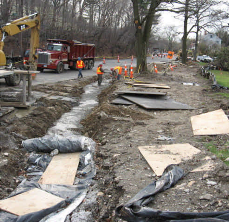
Both photos show trenching activities in the shoulder of Pequot Ave. near its intersection with Rt. 1. Left: Trench is being backfilled; erosion controls should be re-established at the close of each workday. Right: Soil stockpile associated with trenching activities. The pile remained stable and contained after a 1" rain event. Any sections of erosion controls in disrepair should be re-established.
