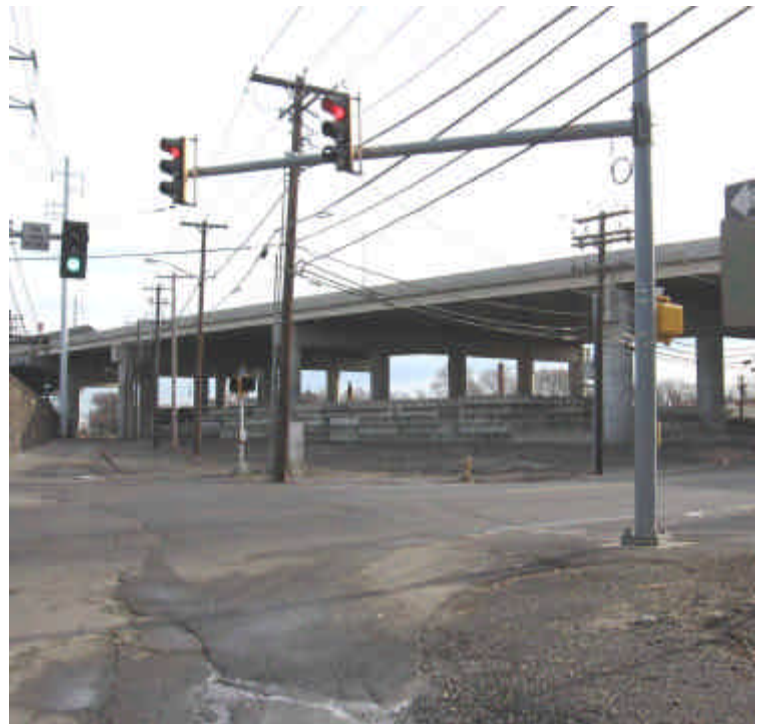
Photograph of the former Iranistan Ave. storage area for the project that has since been abandoned.
