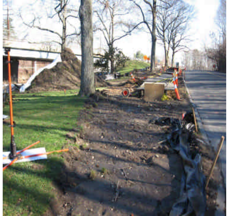
Photo of trenching activities along Pequot Ave. near its intersection with Rt. 1. The silt fence along this area is slumping in some areas. It is recommended that the silt fence be maintained and the plastic covering on the soil stockpile be replaced.
