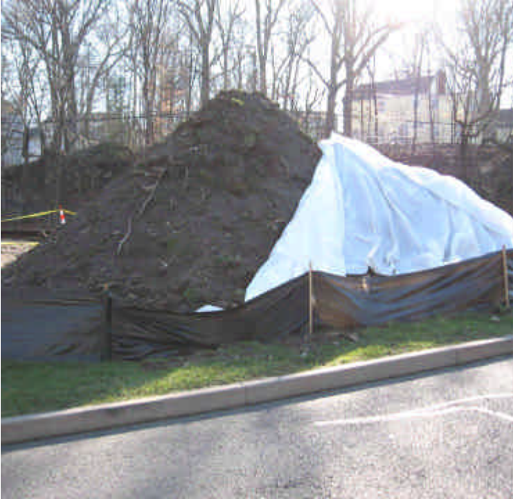
Photo of trenching activities along Pequot Ave. near its intersection with Rt. 1. The silt fence along this area is slumping in some areas. It is recommended that the silt fence be maintained and the plastic covering on the soil stockpile be replaced.
