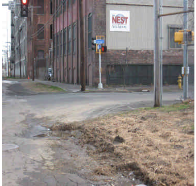
Photograph taken at the intersection of Railroad Ave. and Hancock Ave. of some minor soil migration from the shoulder into the road. Vehicles are tracking soil through intersection.
