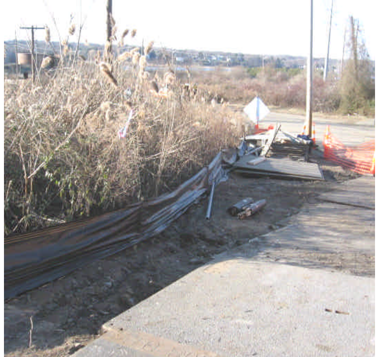
Both photos are of trenching activities from station #1049 to 1051. Resource areas are located immediately adjacent to the trench (indicated by the wetland flagging). Silt fence is installed but was not toed-in and some materials are stored on the opposite side of the controls. Issues in the adjacent areas were not noted but repairs are needed.
