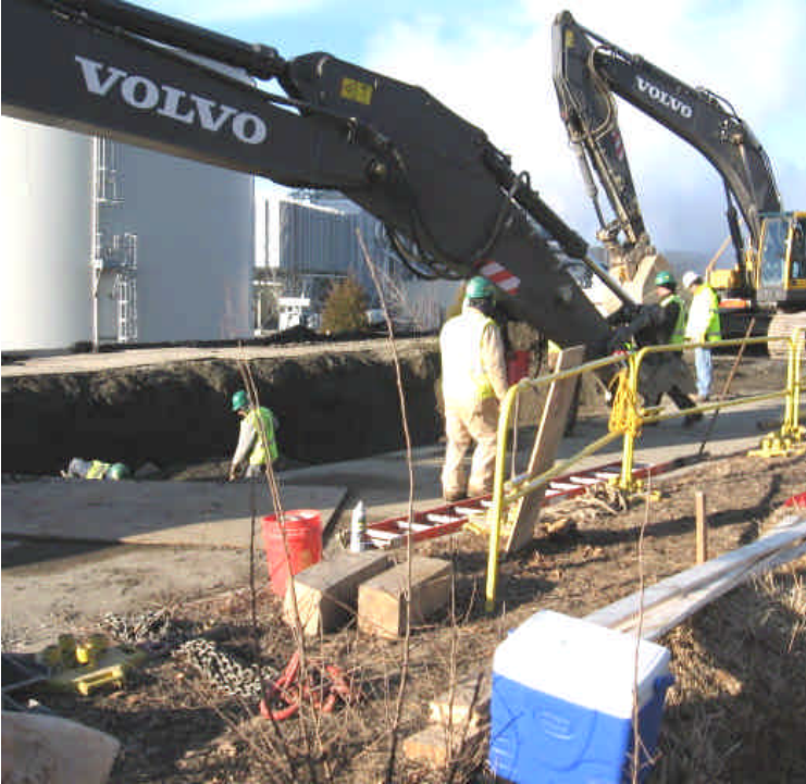
Photograph of Vault #6 installation activities.
