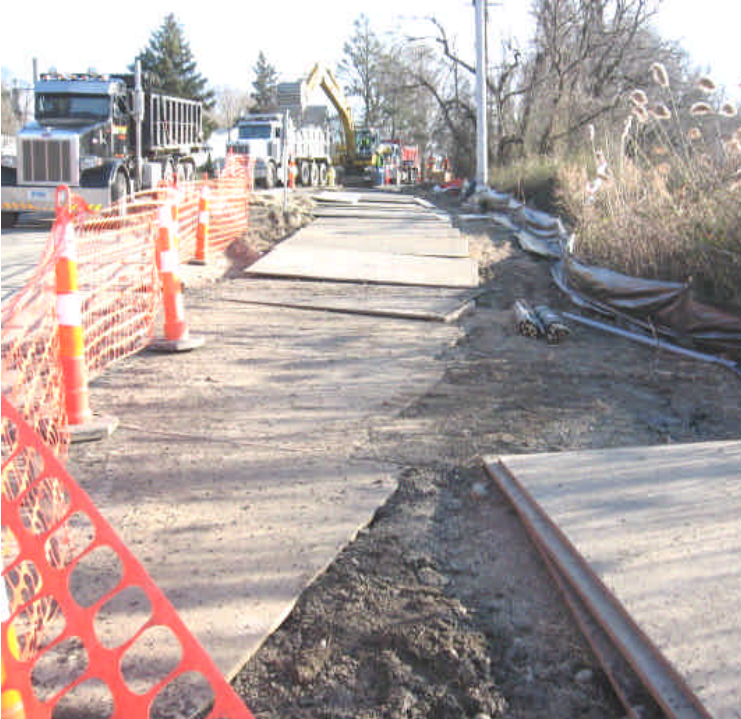
Both photos are of trenching activities from station #1049 to 1051. Resource areas are located immediately adjacent to the trench (indicated by the wetland flagging). Silt fence is installed but was not toed-in and some materials are stored on the opposite side of the controls. Issues in the adjacent areas were not noted but repairs are needed.
