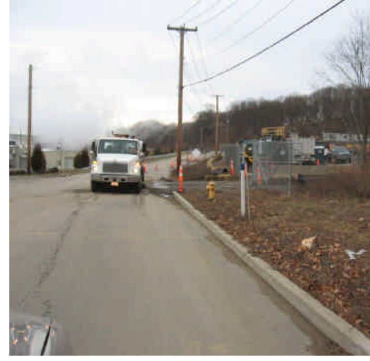
Photo of street sweeping at the entrance to the Millfield lay-down yard. Minor sediment had been tracked onto the roadway.
