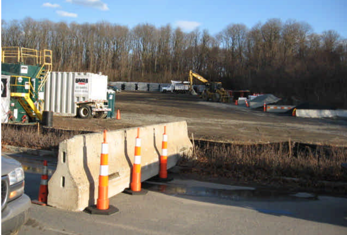
Both photos show the contractor lay-down yard in Milford. Erosion controls surround the entire perimeter of the yard, all loose fill materials are being stored within jersey barriers. The access to the yard has a stone construction entrance to prevent sediment tracking. No issues were noted at the time of inspection.
