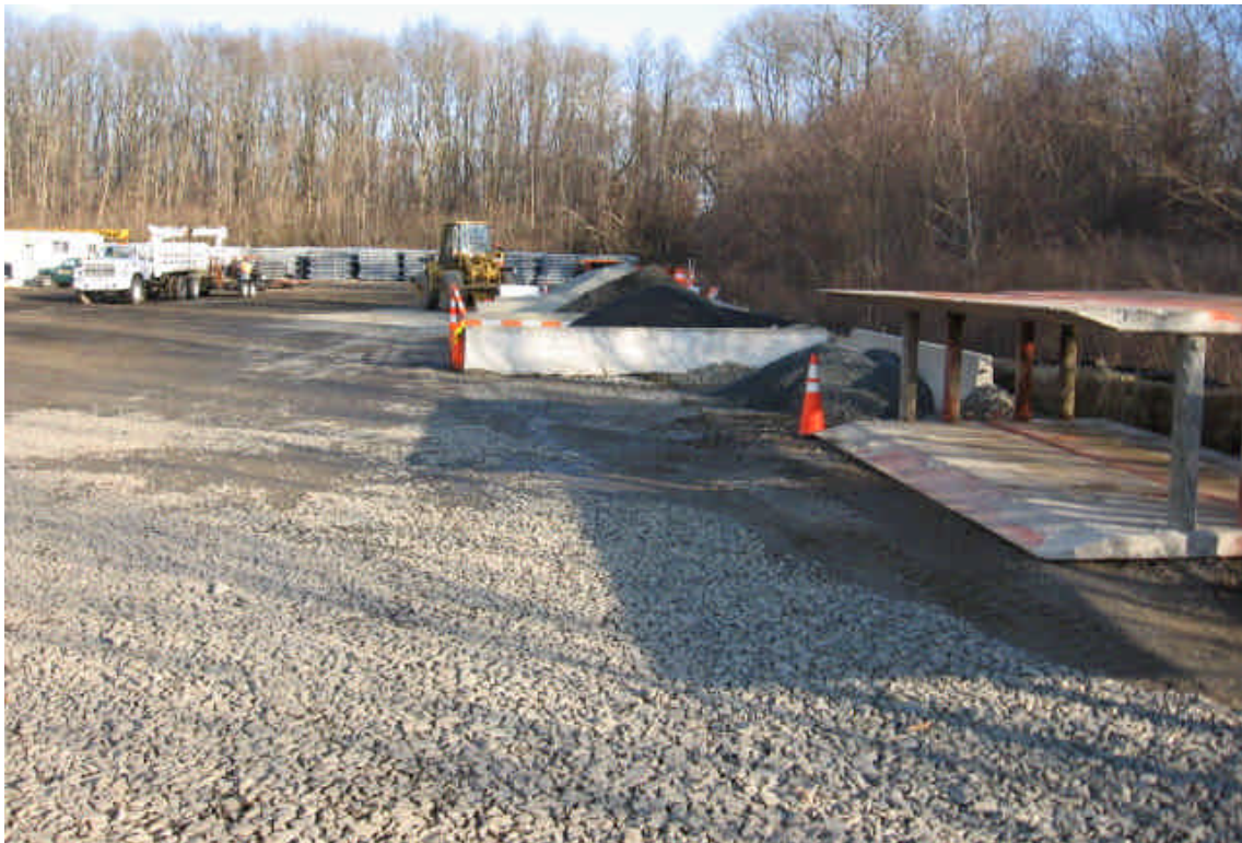
Both photos show the contractor lay-down yard in Milford. Erosion controls surround the entire perimeter of the yard, all loose fill materials are being stored within jersey barriers. The access to the yard has a stone construction entrance to prevent sediment tracking. No issues were noted at the time of inspection.
