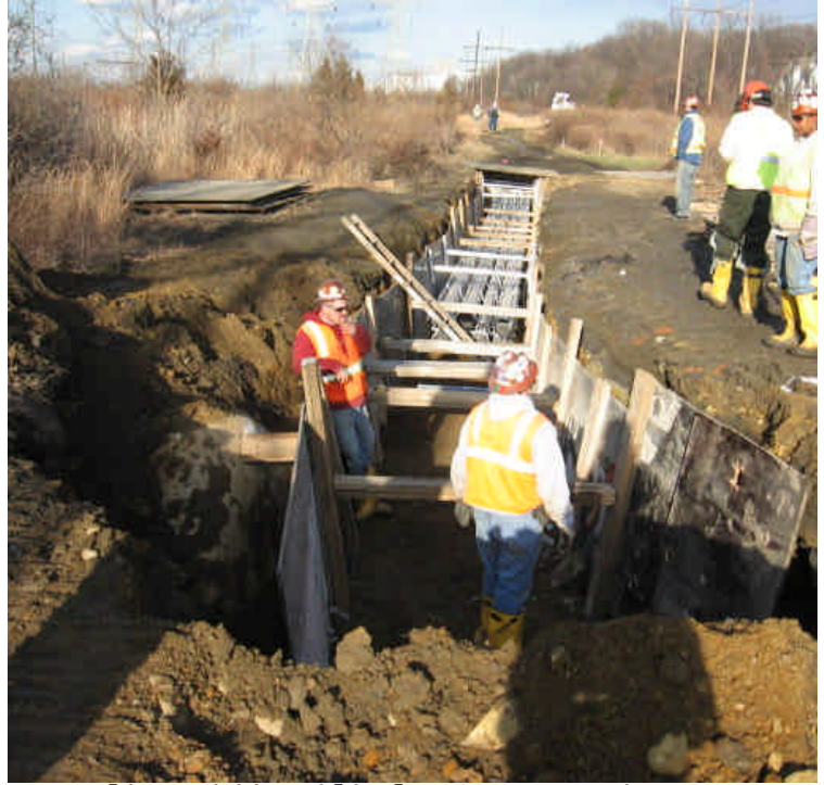
Trenching activities within the ROW near station 1053.
