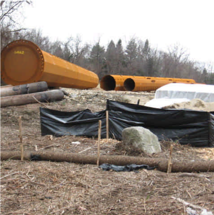
Structures have been delivered for installation off Route 152 (east).
