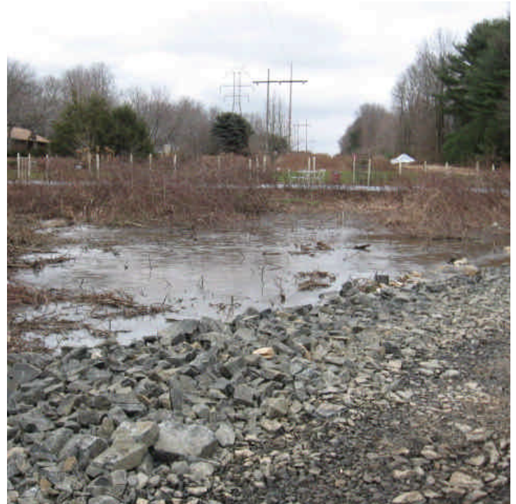
Water continues to pool along the access road within the ROW off Route 152 (west).
