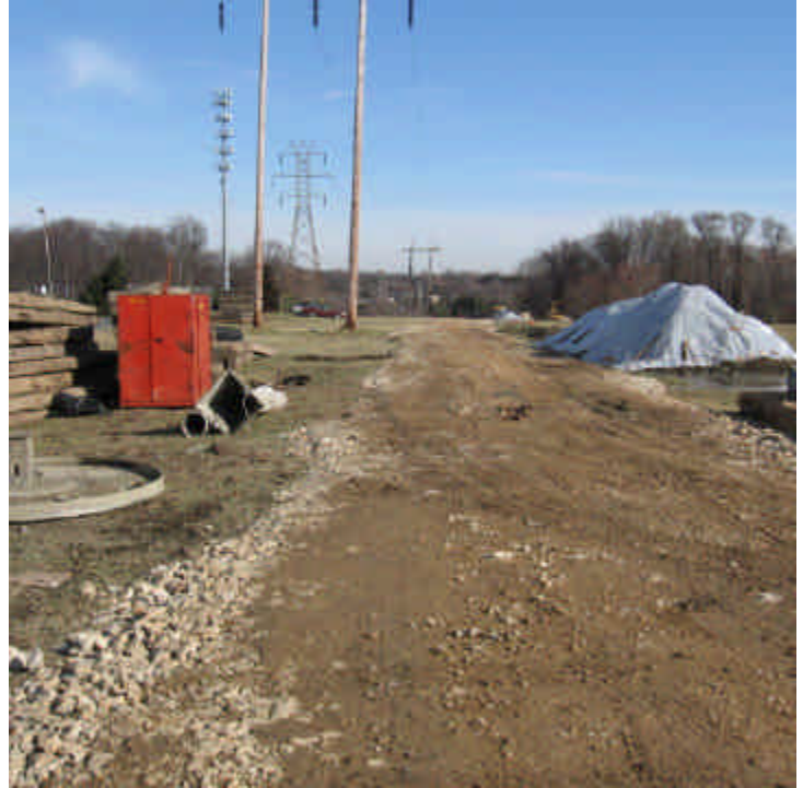
Overall view of the work within the ROW off Route 152 (east).
