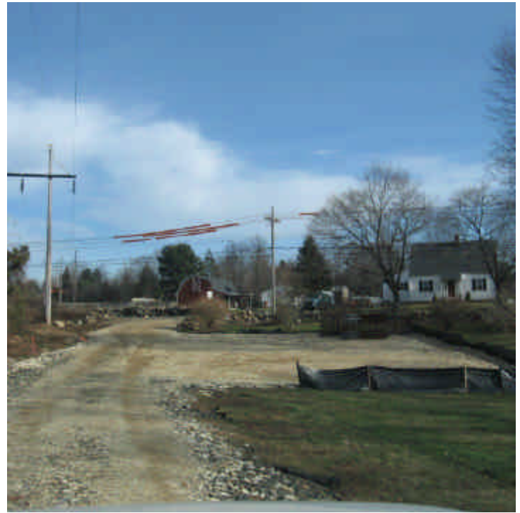
Silt fence remains intact along work areas off Rolling Ridge Rd.
