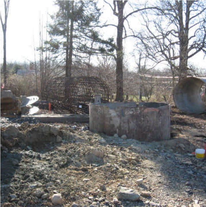
View of the foundation work within the ROW off Dogwood Rd.
