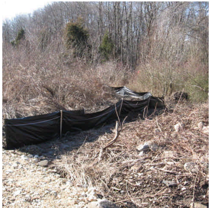
Silt fence remains intact along the wetland boundary off Sunset Dr.
