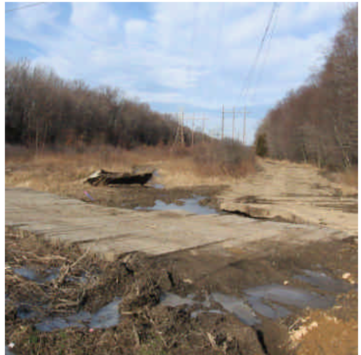
Additional mats were placed along the access road here (Pease Rd).
