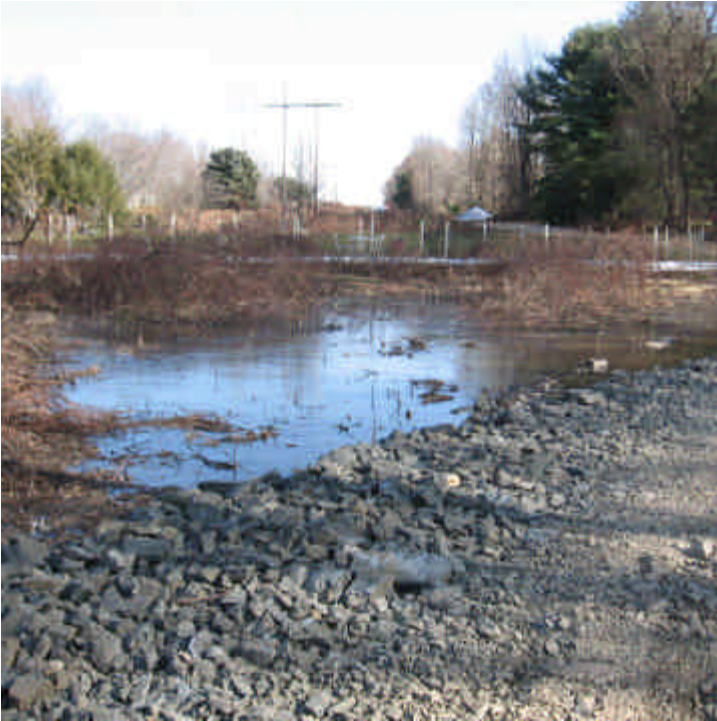
View of the water pooling at the access road located across from the wetland area off Route 152 (west). Additional stone could be placed in the access road here to reduce vehicle tracking/turbidity.
