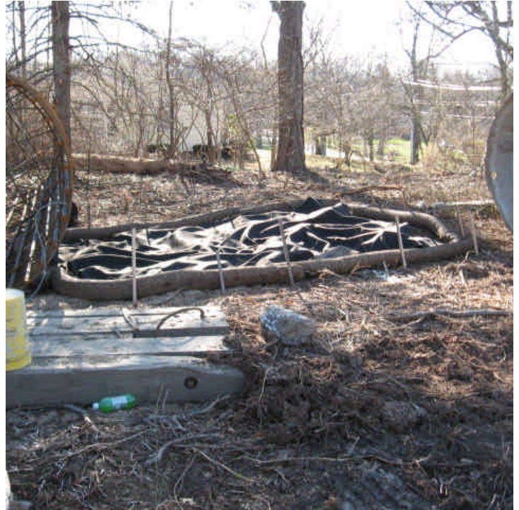
Dewatering controls were installed proactively off Dogwood Rd.
