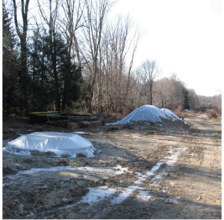
Overall view of the work within the ROW off Route 152 (west).
