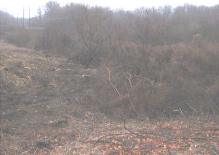
View of the clearing within the ROW located off Lexington Lane (east) in Milford. Continue to retain shrubs whenever feasible.
