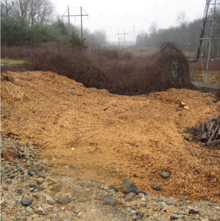
View of the wood chips pile within the ROW off Hunting Hill Place. Wood chips are currently at a depth greater than 3" and should be spread in upland areas or removed.
