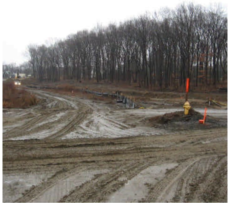
Activities associated with the relocation of Shelland Street continue in Milford.
