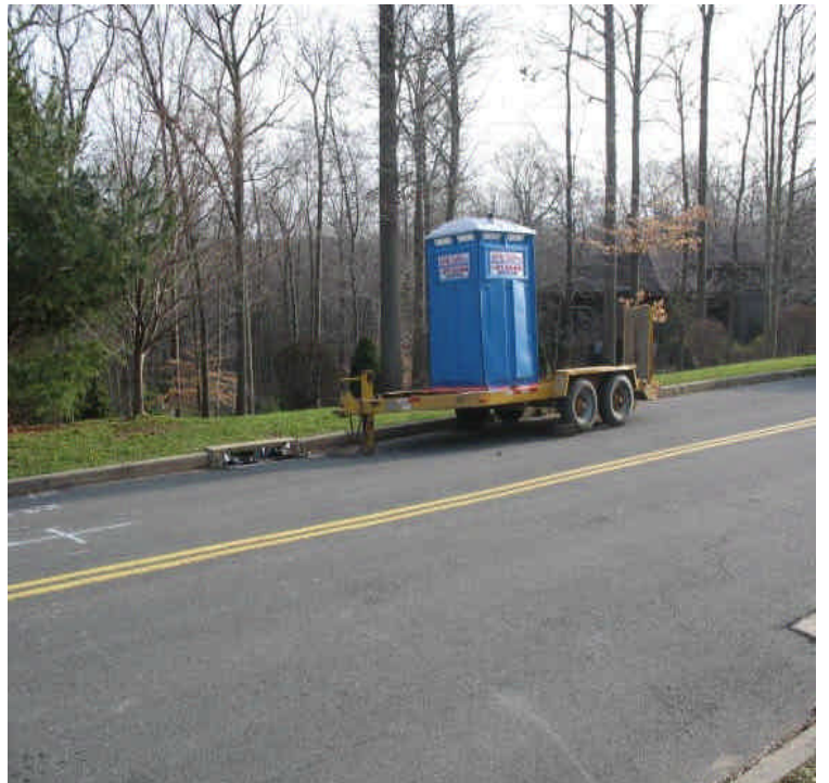
Portable sanitary facilities should be moved away from wetlands and catch basins to reduce the potential for impacts.
