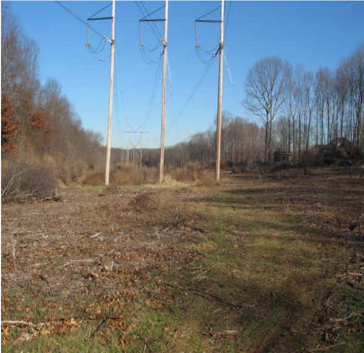
ROW off Stony Brook Rd. Non-project related debris had been dumped near this area.
