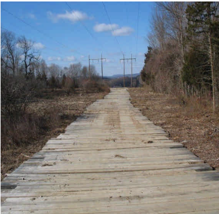
Access road (timber mats) in place off Haddam Quarter Rd.
