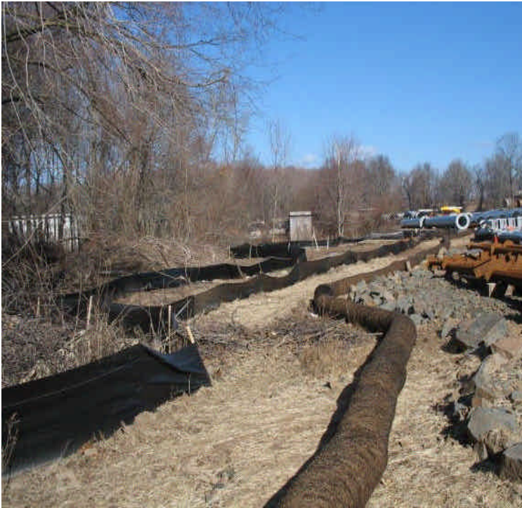
Additional controls remain in place adjacent to wetlands to filter/contain any turbid run-off leaving the site.
