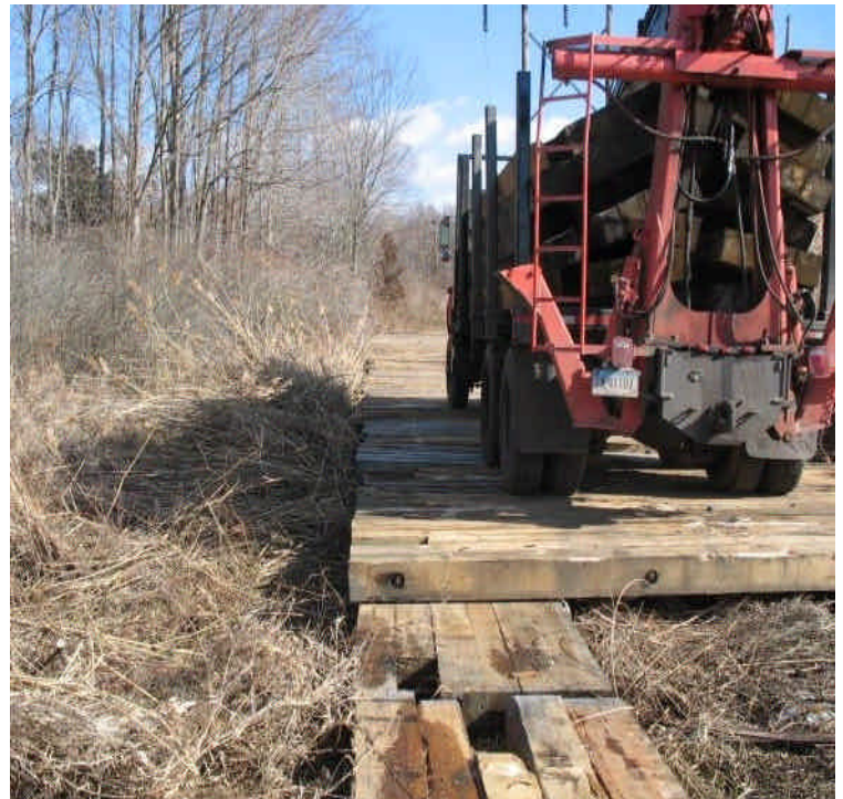
Timber mat installation off Durham Rd. Erosion controls may be needed.
