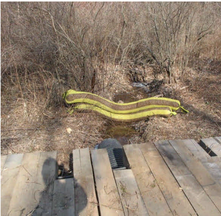
View of a timber mat crossing over a small stream in the wetlands located west of Powder Hill Rd. Filter socks were added for control of potentially turbid run-off. No sediment was noted leaving this area.
