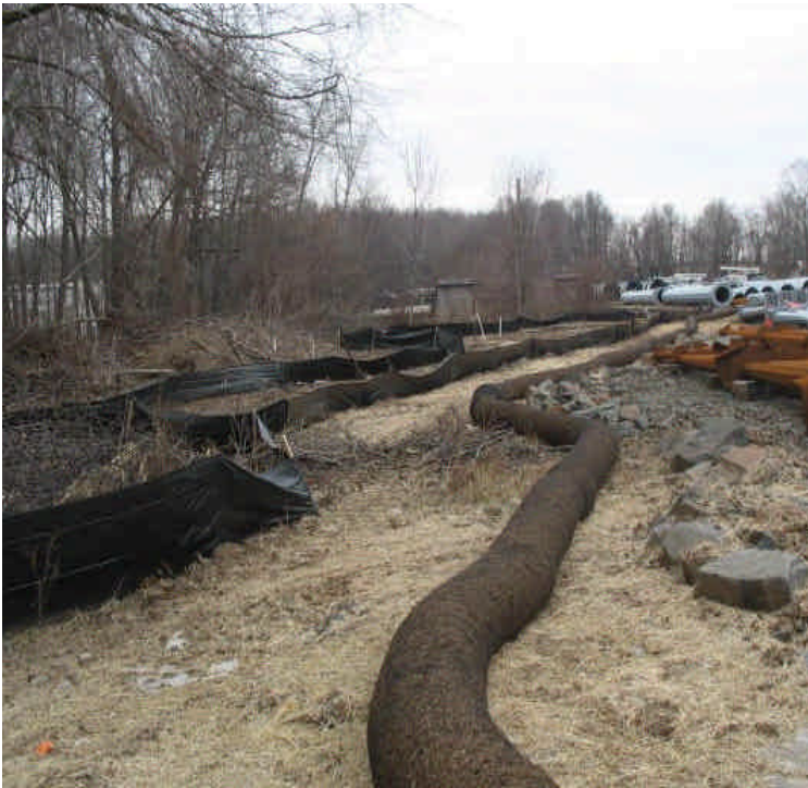
Additional controls remain in place adjacent to wetlands to filter/contain any turbid run-off leaving the site.
