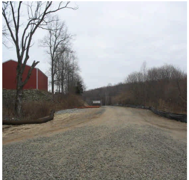
Silt fence, fiber rolls, and hay mulch have been added upgradient of wetland areas adjacent to the contractor receiving yard.
