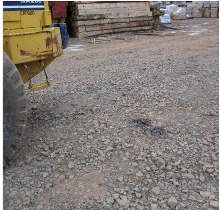
Small stains were noted around the contractor receiving yard including near a leaking forklift.
