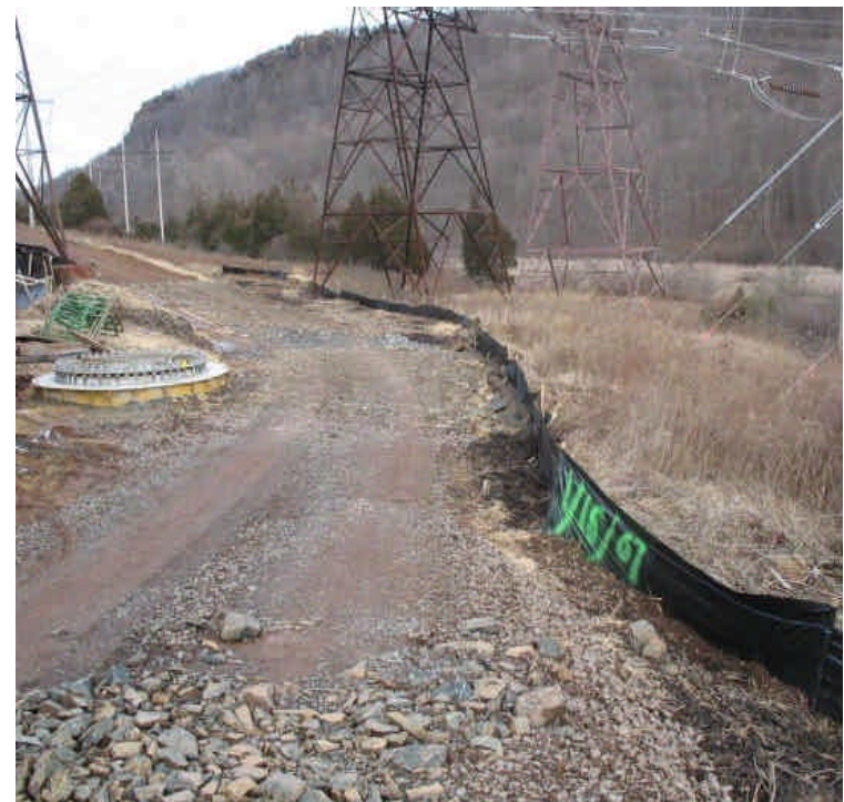
Silt fence extension located upgradient of the wetlands at Black Pond
