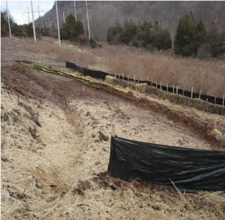
Overview of the haybales, silt fence, and filter socks at Black Pond. Mulch remains in place around the site for increased stabilization.
