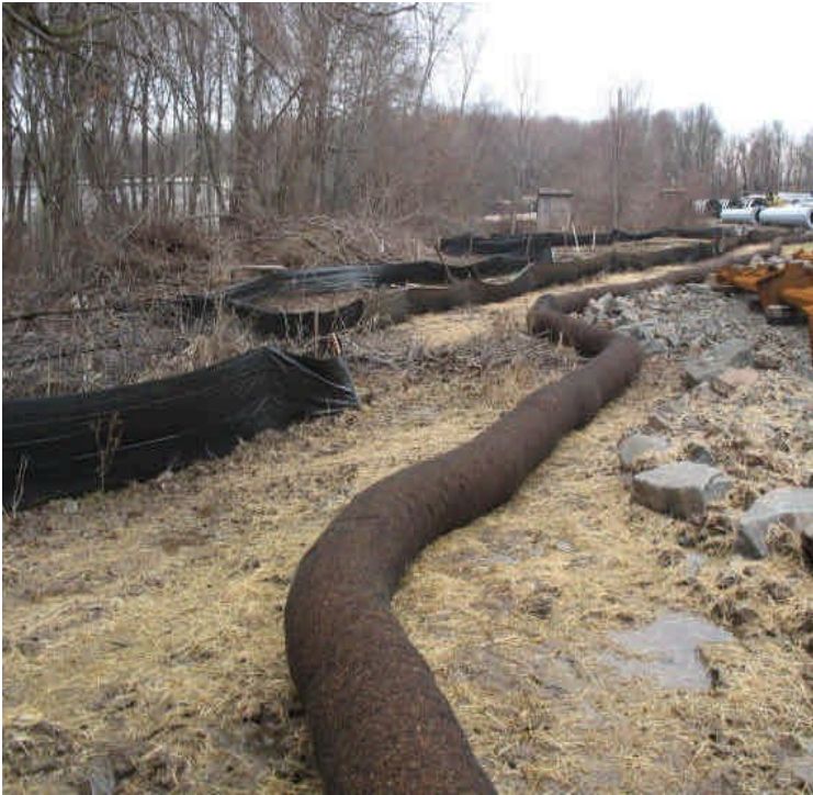
Additional controls were added adjacent to wetlands to filter/contain turbid run-off leaving the site.
