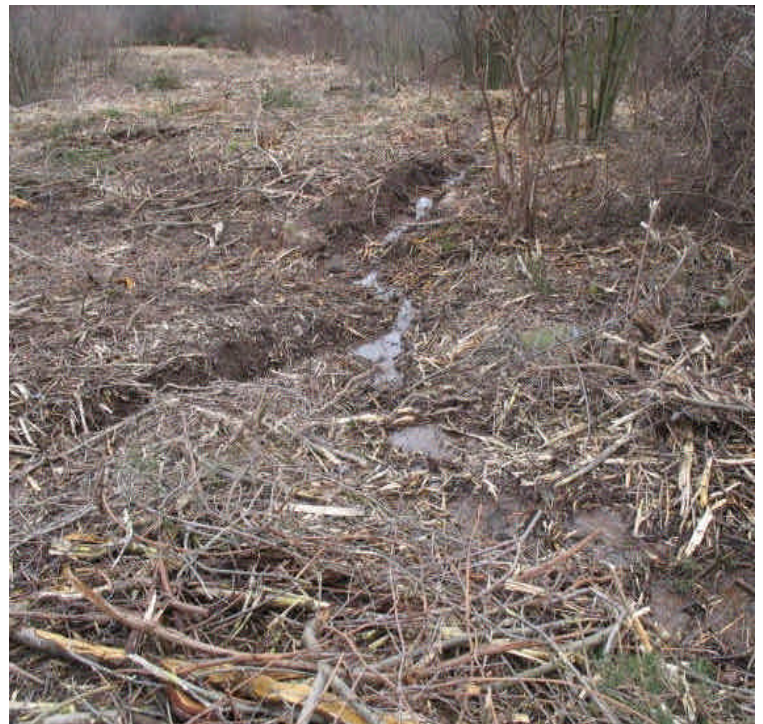
Saturated slope east of Powder Hill Rd within the new clearing. Monitor slope for erosion and changes to run-off patterns. Soils appear stable.
