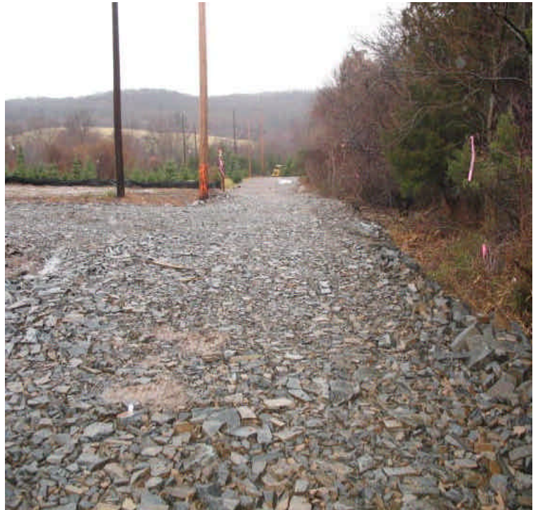
New access road and pad construction east of Powder Hill Rd.
