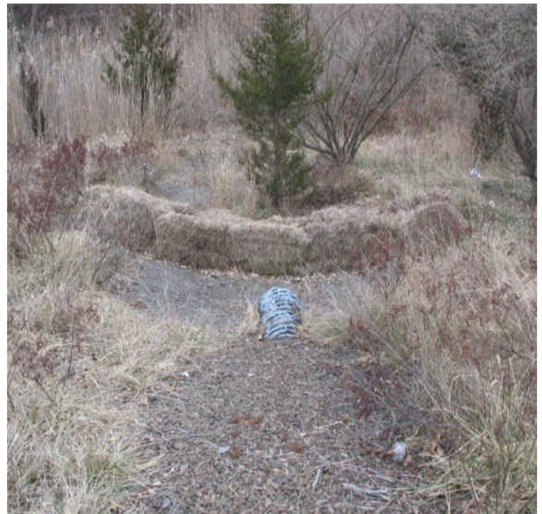
Remove degraded haybales when feasible. Site is stable.
