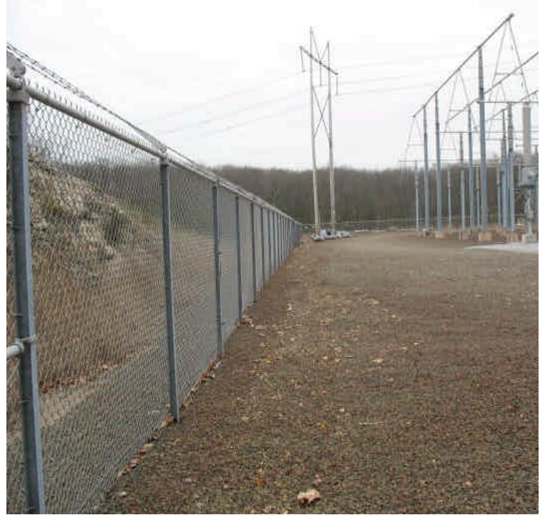
View of the perimeter of the yard. The site is stable and soil disturbing work is now complete.
