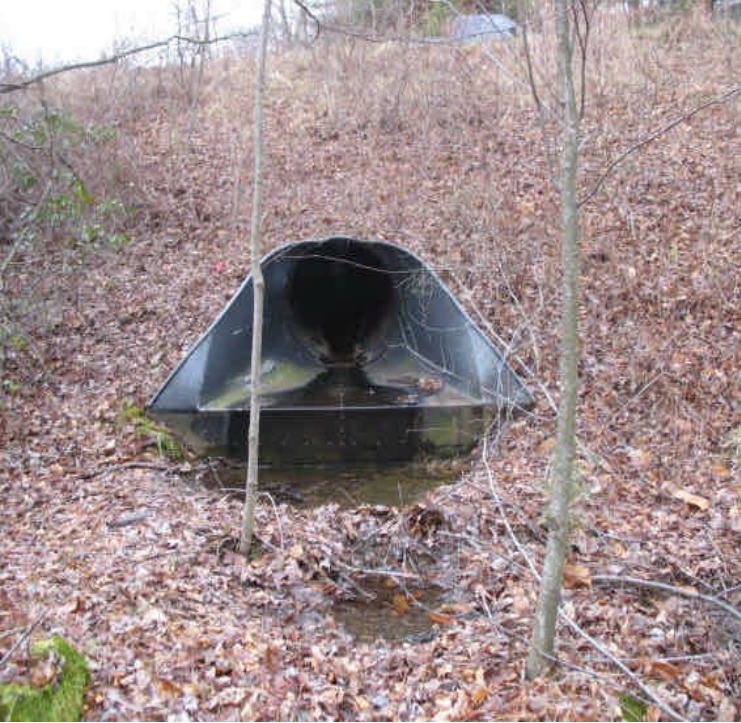
View of the culvert under the access drive. No sediment issues have been observed.
