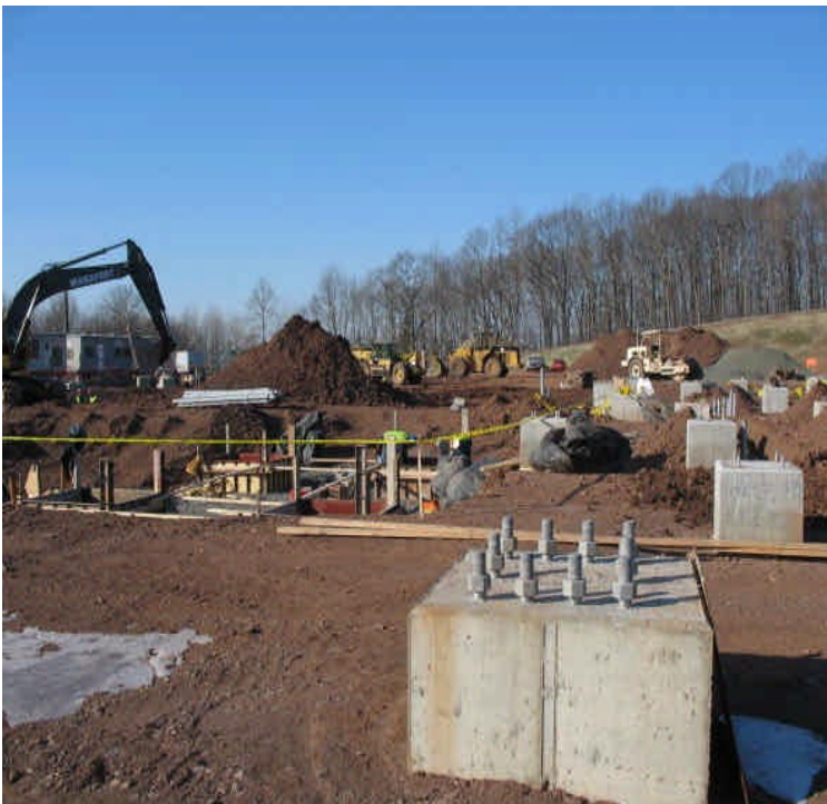
View of foundation installation looking east to west across the site.
