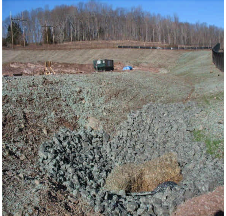
View of the culvert under the new access road. A minor amount of sediment was noted but appears well contained within the trap. Beseck and Seg. 1A contractors are jointly sharing the access road.
