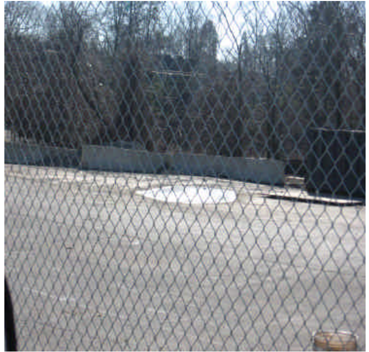
Imperial Ave. lay-down yard was locked at the time of inspection. No issues were noted.
