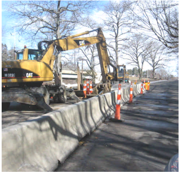
Trenching activities continue along Pequot Ave.
