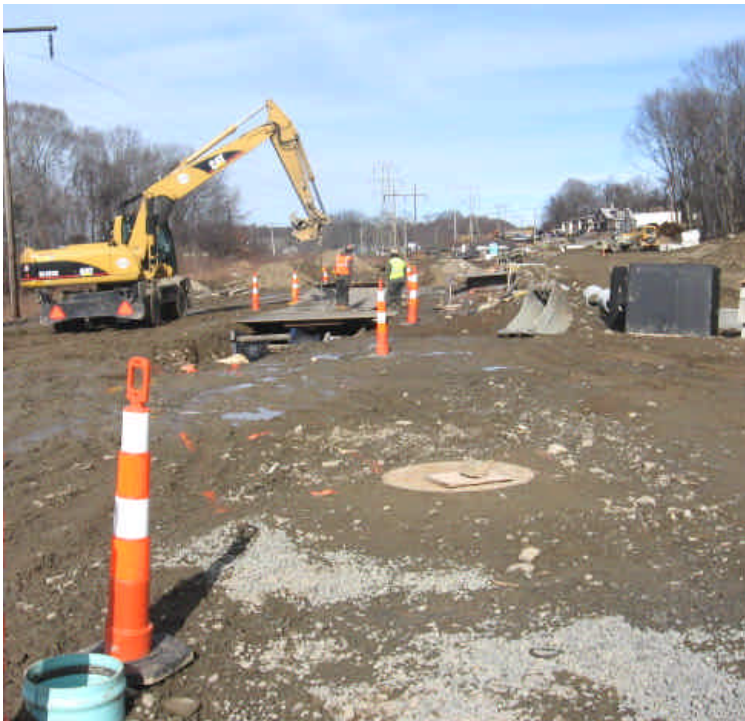
View of the trenching activities being conducted between stations #1110 to 1112.
