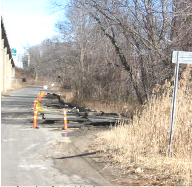
Photo of trenching activities from station #1016 to 1020.
