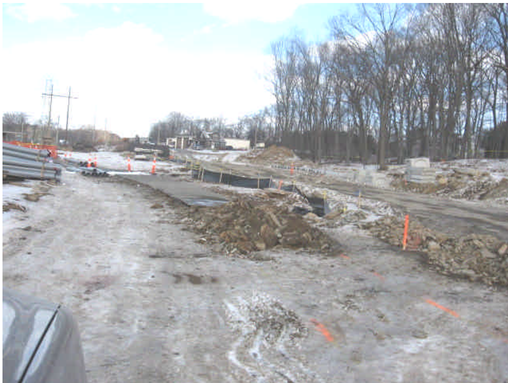
Photo of trenching activities from station #1112 to 1113. No issues were noted.
