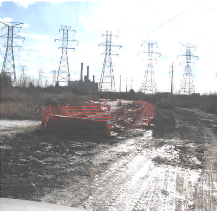
Photo of trenching activities from station #1058 to 1061.
