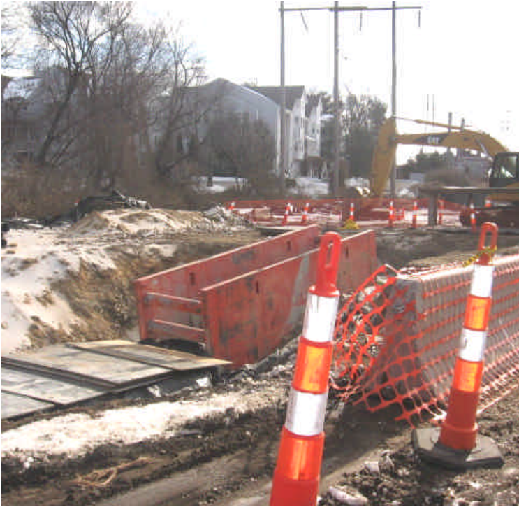
Photo of trenching activities at Vault #4.
