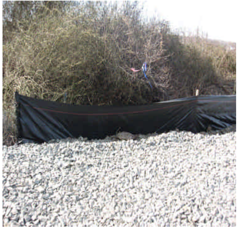
Silt fence has been re-established/repared where necessary along the project route.
