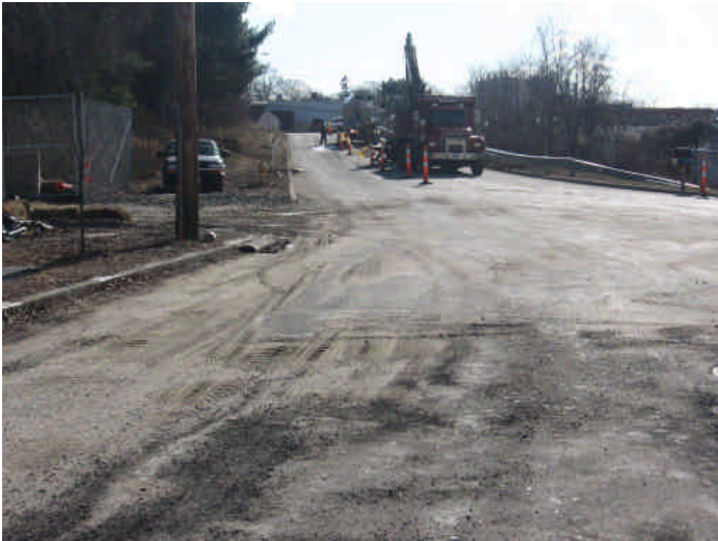
Photo of the entrance of the Milford contractor lay-down yard. It appears that roadway sweeping is occurring, some sediment accumulation remains near the curbing or gutter. This may need to be removed by hand if sweepers can't reach it.
