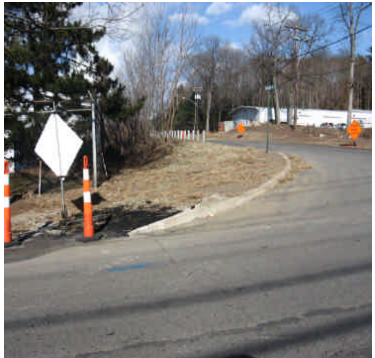
Exposed soils on the corner of Shelland and Caswell Sts. have been temporarily stabilized with hay mulch.
