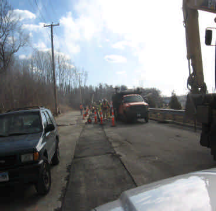
Both photos show a view of trenching activities along Shelland St. All catch basins have been adequately protected with controls.
