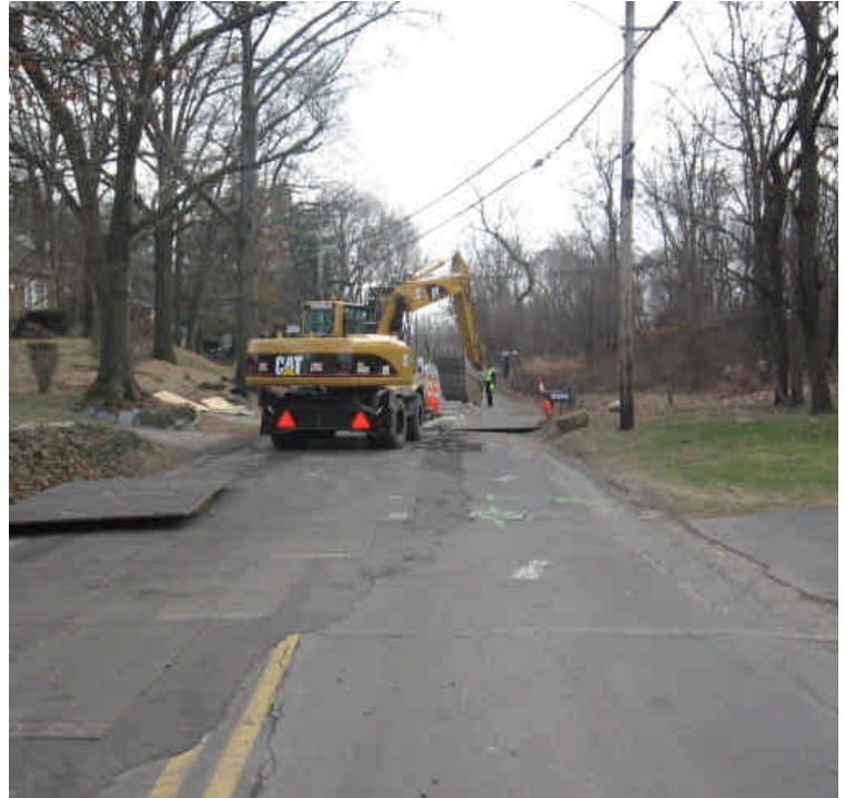
View of trenching activities in the roadway near station #1035.
