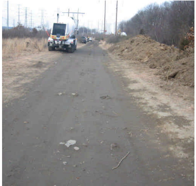
Construction access road has been watered down for dust control.
