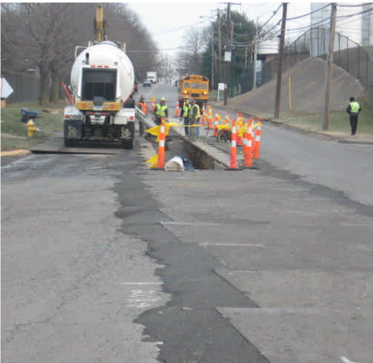
View of trenching activities in the roadway at station #1081.
