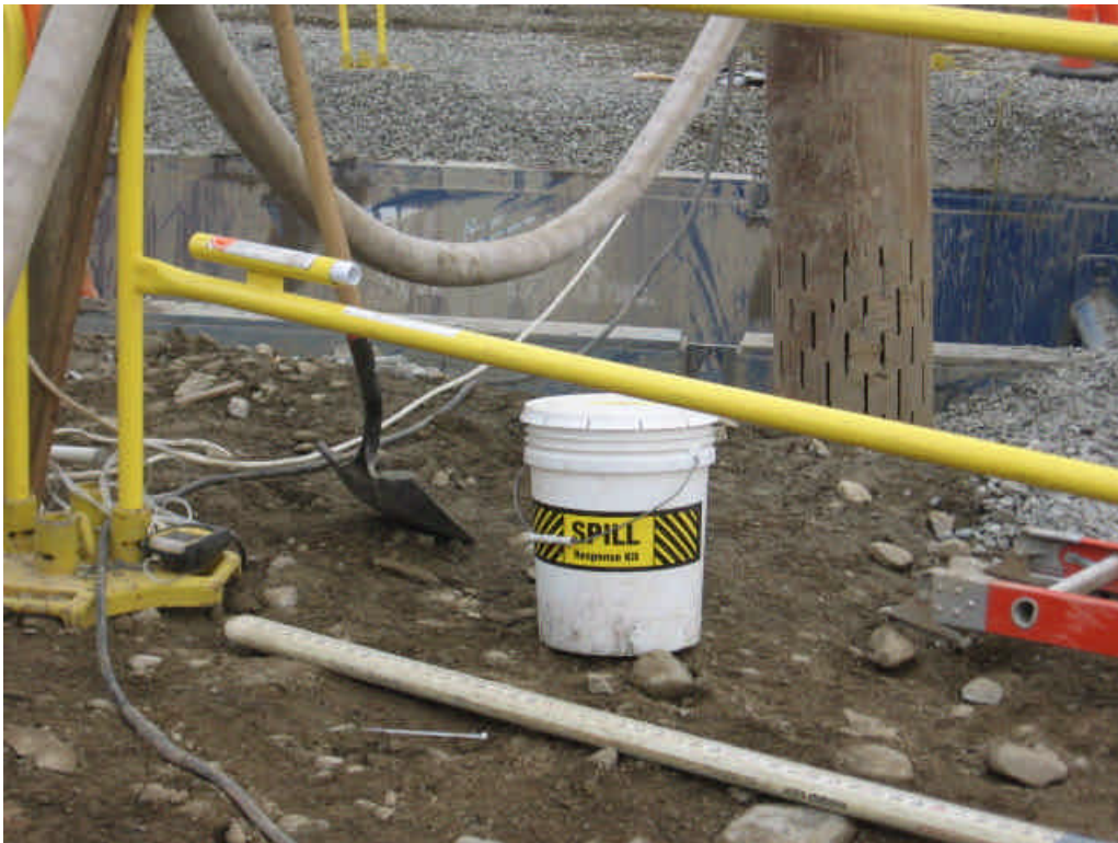
Above: Photo of Vault #7 installation activities. The adjacent construction activities are not covered by the Segment 3 inspection. Below: Photo shows a spill kit that was observed on site with the vault construction. Continue to be proactive about bringing these materials to active sites.
