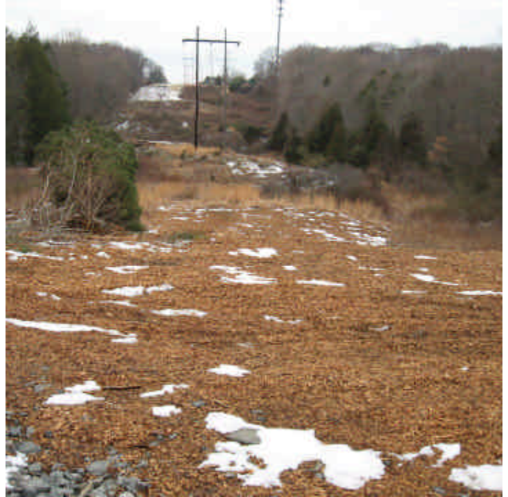
Wood chips were spread appropriately within the disturbed upland portions of ROW off Lambert Rd.
