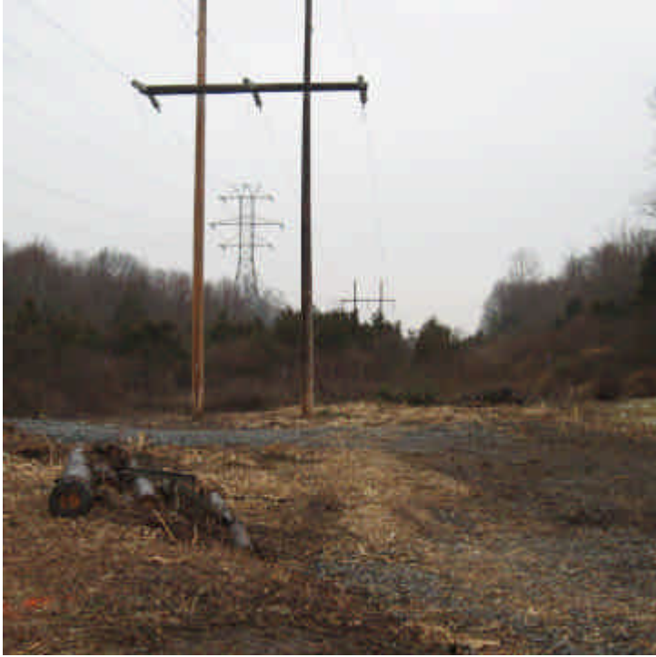
View of the clearing and access road construction off Salem Road.
