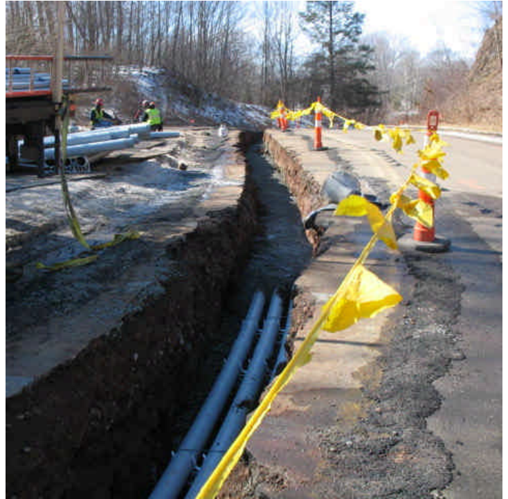
Trenching conduit installation and backfilling continues within Old Lane Road.
