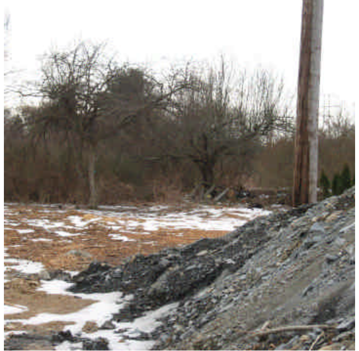
Wood chips were spread in the disturbed areas adjacent to the wetland off Hall Drive.
