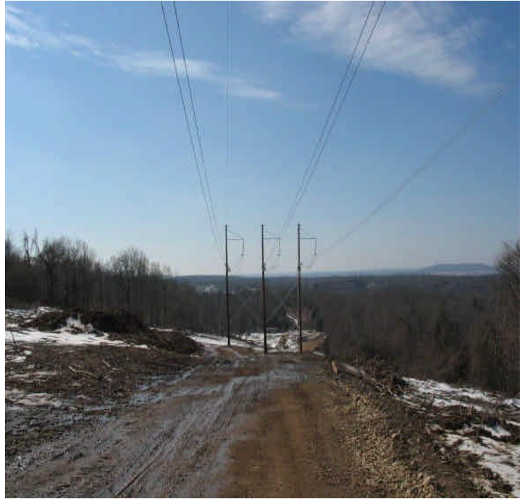
View of the staging areas. Poles/line installation complete in this location.
