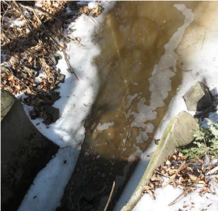
Turbid run-off was flowing into the CBs along Old Farms Rd. and was observed entering the adjacent wetlands. Liners were in place but gutter buddies had been removed and needs to be restored.
