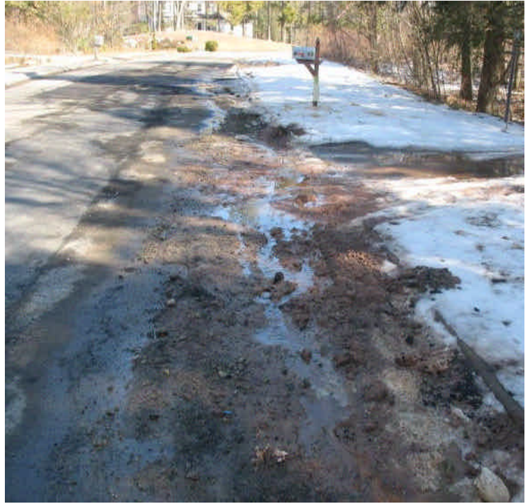
View of sediment accumulation along the gutter near a catch basin along Old Farms Rd. Gutter buddies were not in place, likely due to town plowing. Sweep by hand if the street sweeper cannot reach this
