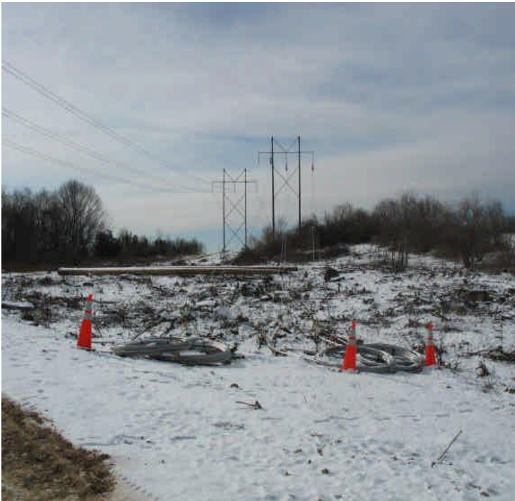
View of poles installed and wires pulled off High Hill Road.
