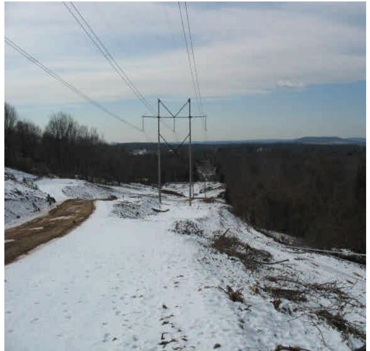
View of the staging areas. Temporary stabilization measures (mulch) are added as needed.
