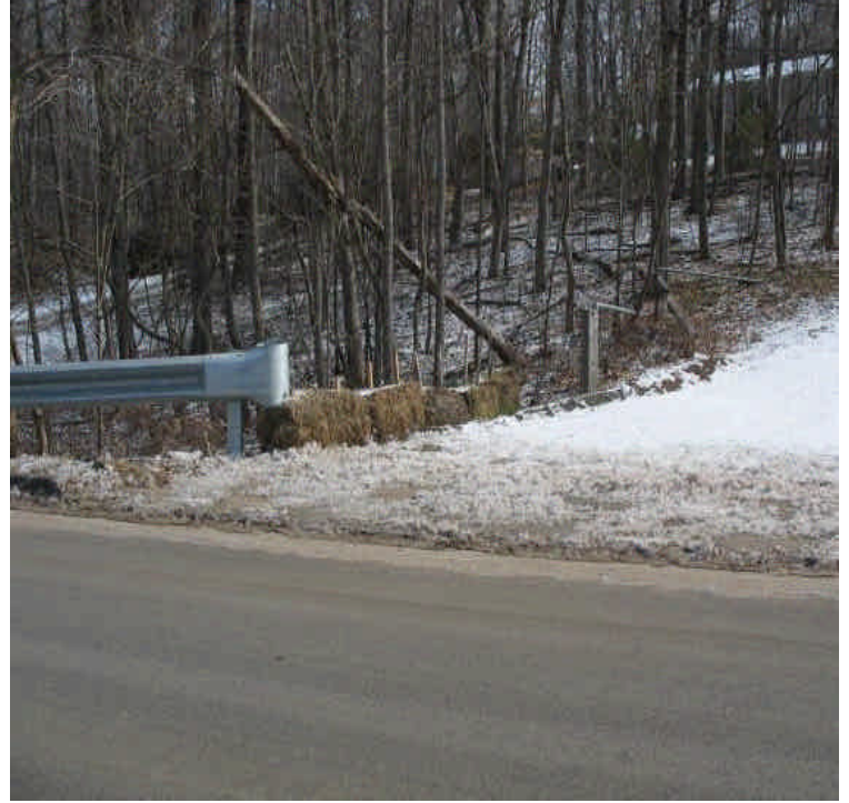
Silt fence removed at the ROW access off Mansion Rd. No erosion issues noted.
