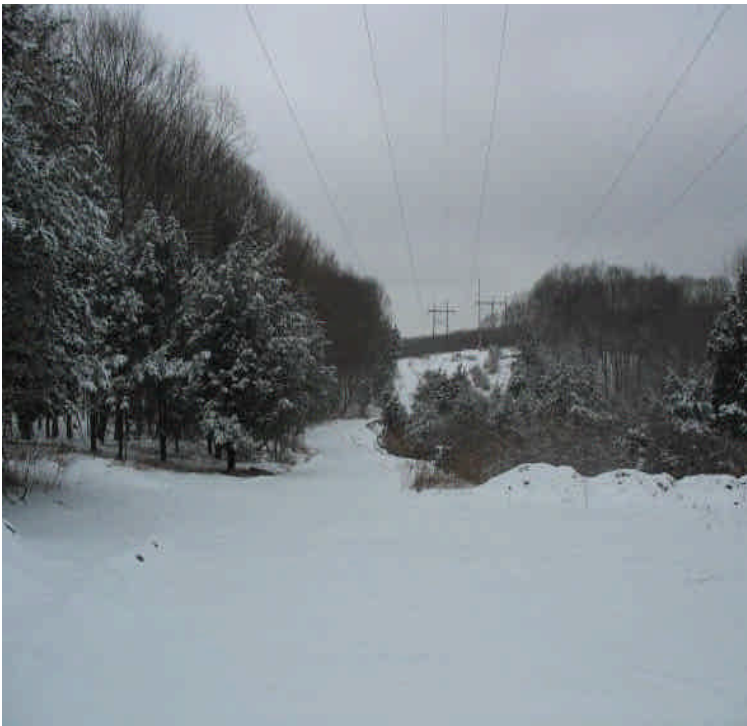
Timber mats in place for access west of Arbutus Street. No run-off was noted during the inspection.
