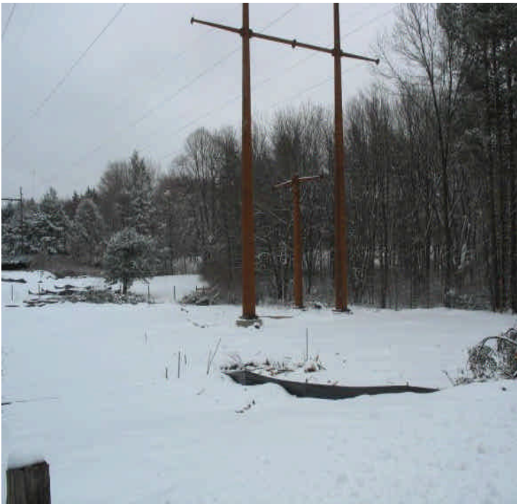
Foundations and poles installed along ROW between Little Lane and Route 17.
