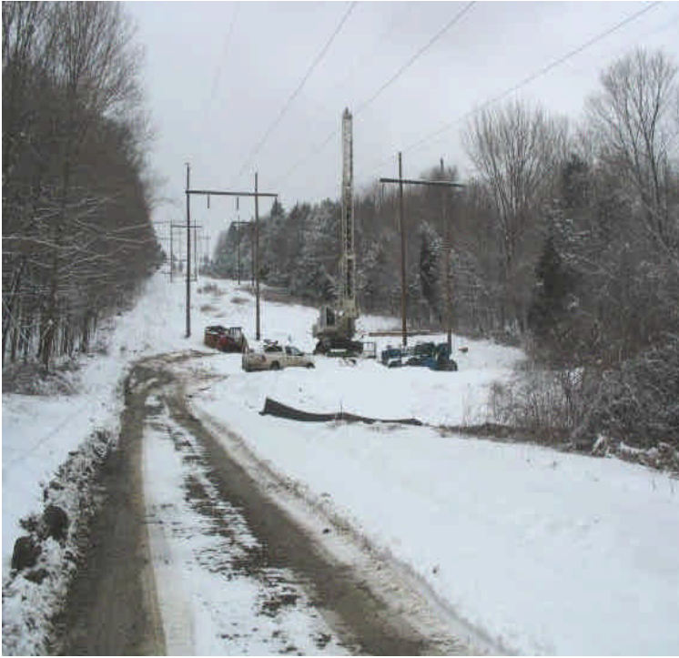
Both photos show foundation drilling west of Powder Hill Rd. No active dewatering was noted during the inspection. Controls were in place downgradient.
