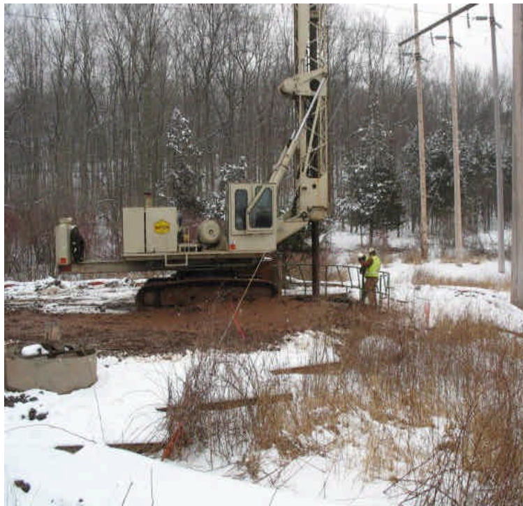
Foundation drilling along the ROW east of Beseck SS. Controls were in place to prevent sediment from entering the wetlands.
