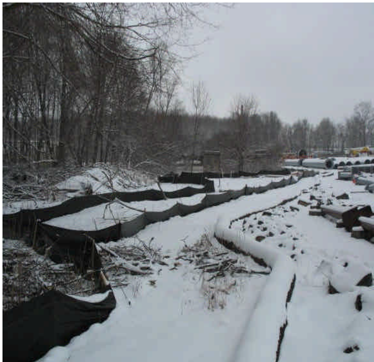
Additional controls remain in place adjacent to wetlands to filter/contain turbid run-off leaving the site.
