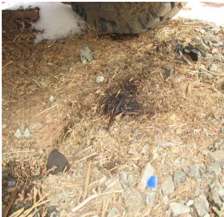
The same piece of leaking equipment was noted off Powder Hill Rd from last inspection. The spill pads were removed but adequate containment was needed. Repair the equipment as soon as possible.
