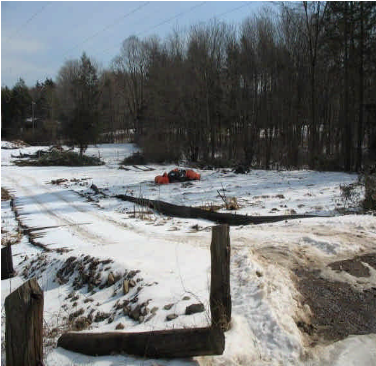
Foundations installed last week along ROW between Little Lane and Route 17.
