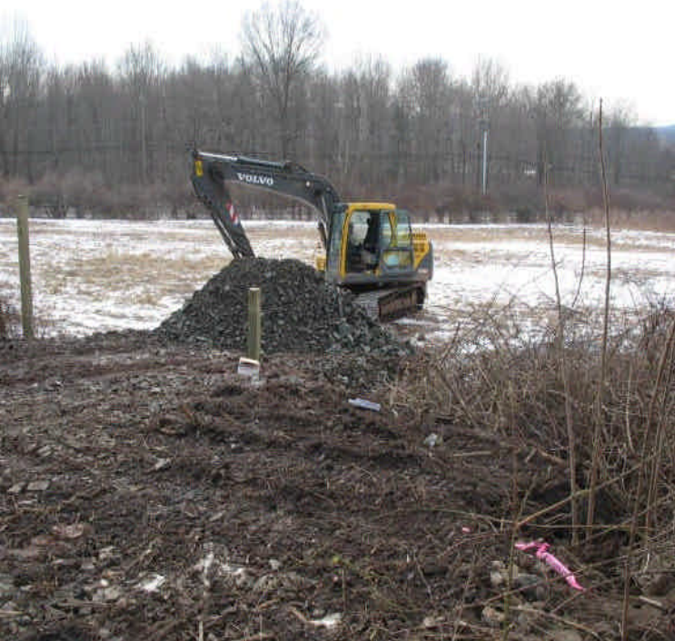
New access road construction off Durham Rd.
