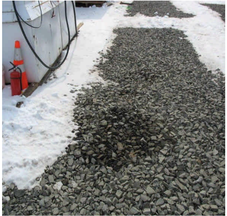
The fuel storage tanks remain in place on the stone spill pad and nozzles are contained. Small drip stains are noted and are contained to the stone.
