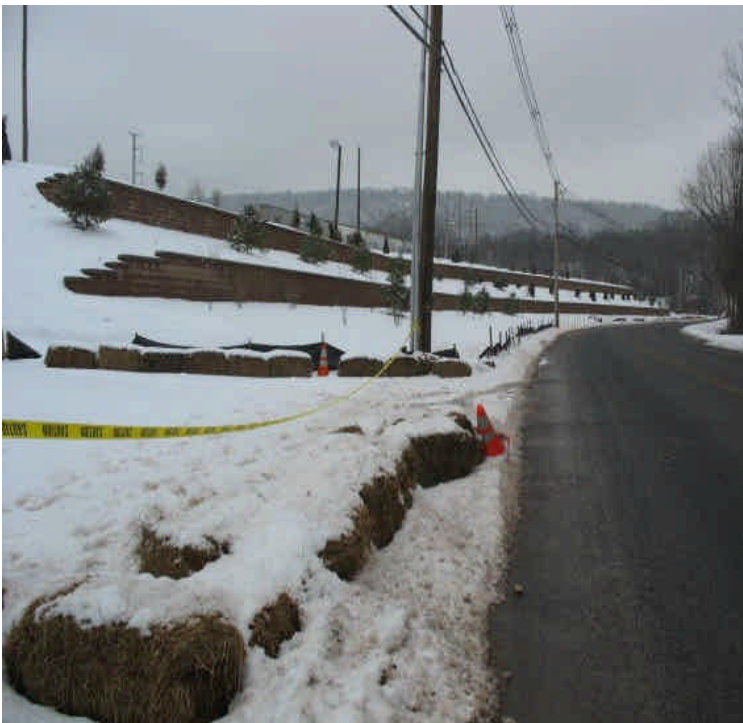
Haybales were placed across the closed site entrance (west side) in an effort to reduce turbid run-off from the site. A small detention area was also constructed. Snow cover also helps to stabilize the area; continue to monitor during thaw periods.
