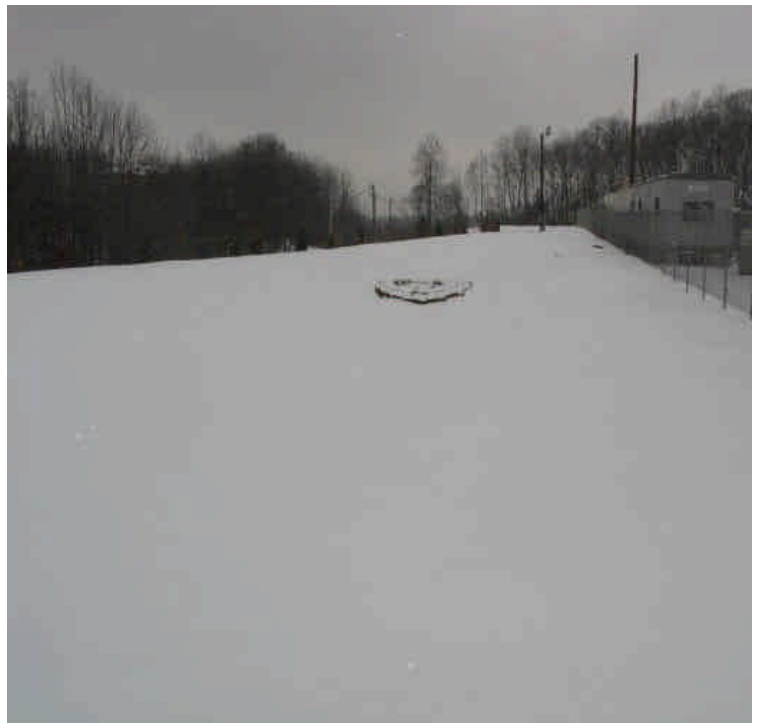
Surface areas on site are temporarily stabilized with snow cover. Haybales and controls remain in place at the inlet of the detention basin.
