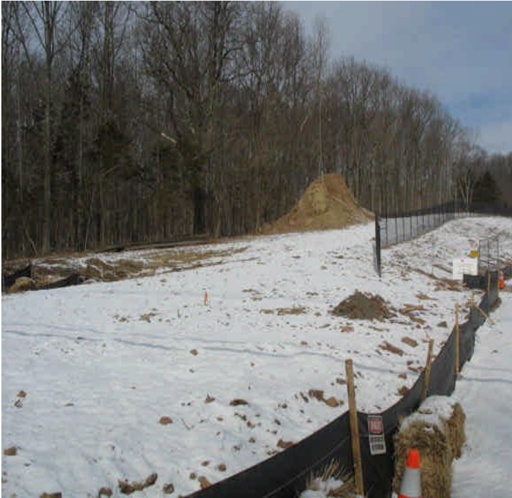
Haybales were placed across the old Zolnik driveway. The remaining stockpile and exposed surfaces are temporarily stabilized with hydro-seed and as a result of freezing temperatures.
