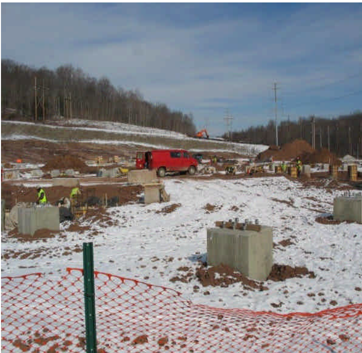
View of foundation installation looking south to north across the site.
