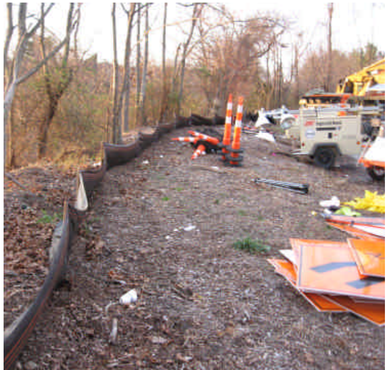
Both photos are of the new laydown yard in Westport on Imperial Ave. The yard is located immediately adjacent to the Saugatuck River on the southwest, west, and north sides. Erosion controls are in place around the perimeter of the yard, adjacent to the river.
