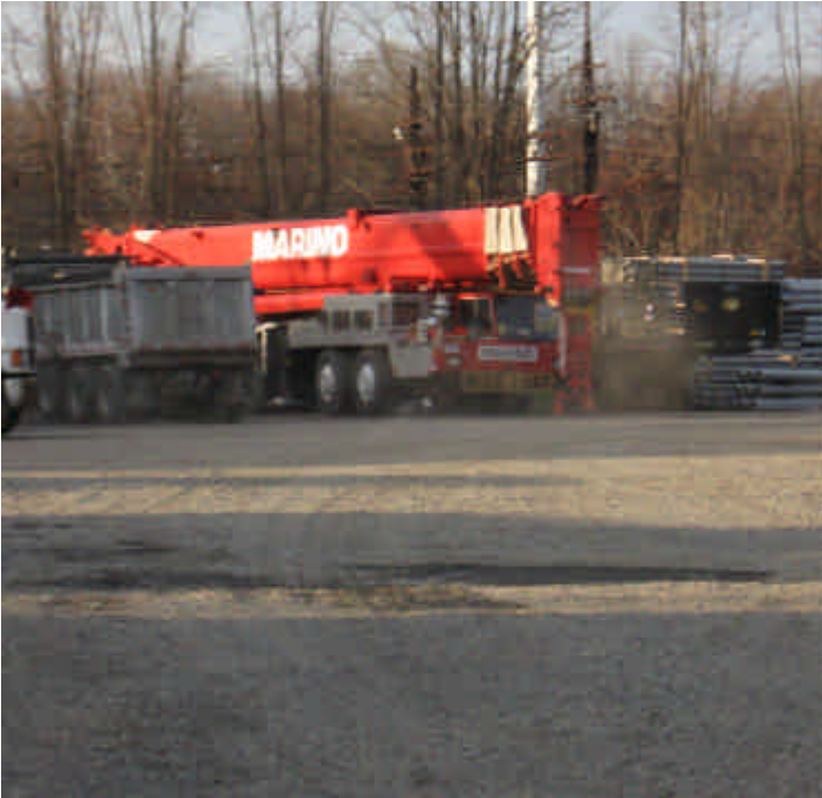
Some airborne dust was noted in the yard during vehicle movement. Evaluate methods to control dust if necessary since the last inspection.
