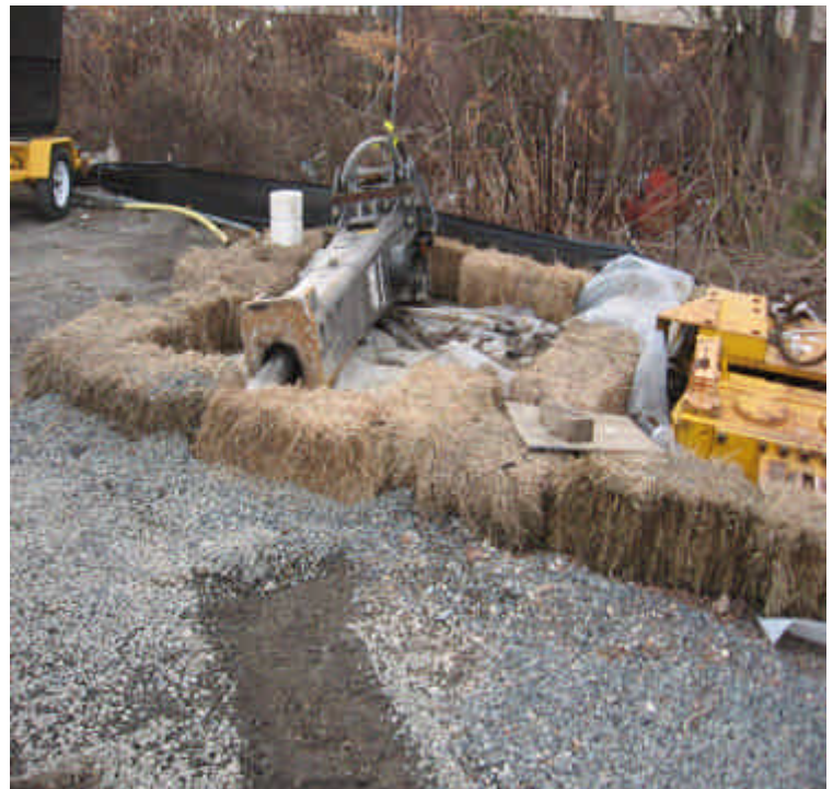
Equipment attachment storage area has now been fully enclosed with controls as recommended.
