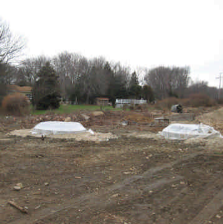
View of the foundation work within the ROW off Russell Ave.
