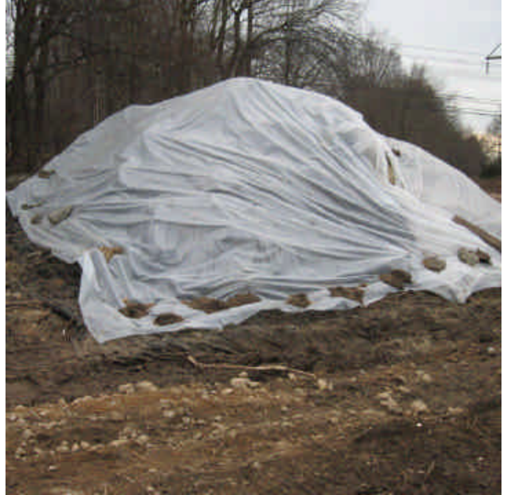
All stockpiles off Russell Ave remain covered with plastic.
