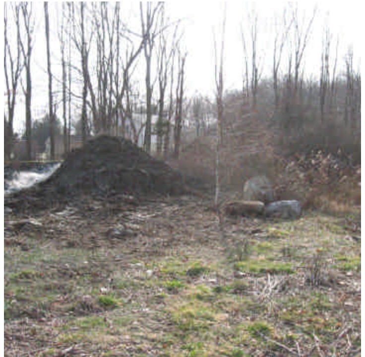
The spoil pile located off Overland Drive (west) is currently stored near the wetland. Silt fence should be installed here.
