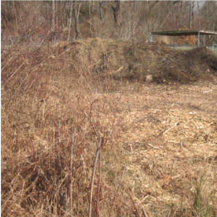
Wood chips were spread along the upland portions of the ROW off Sunset Dr. Take care to keep wood chips out of wetland areas.
