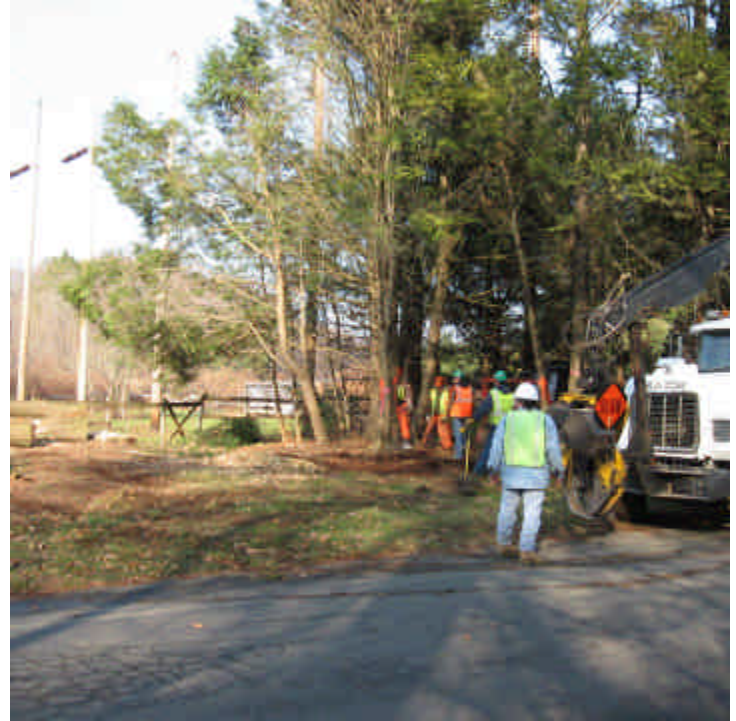
Clearing has begun in the ROW located off Ridge Road.
