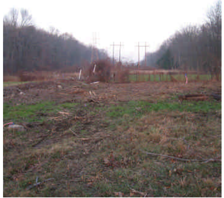
View of the wetland area located just beyond the third structure off Russell Ave.
