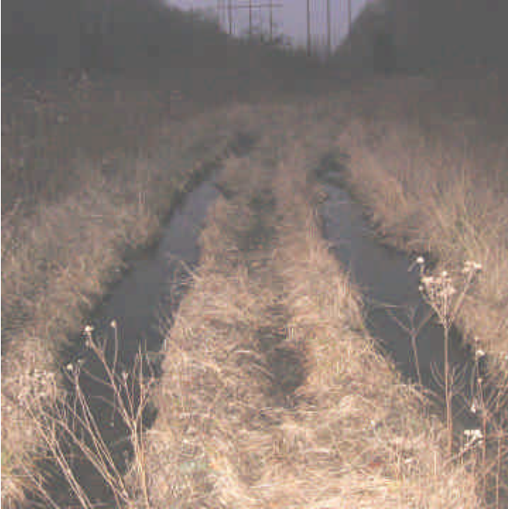
View of the wetland area located within the ROW off Pease Road in Milford. Vehicle tracks were observed within the wetland here. It is unclear whether this is project related.
