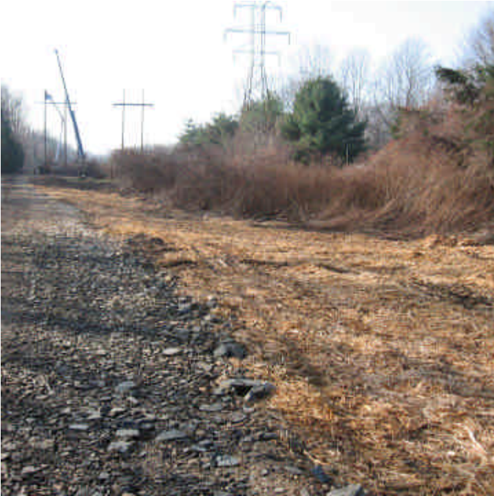
View of access road constructed off Route 152 (west). Wood chips have been spread within the ROW here.
