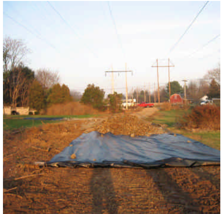
Access road construction continues off Rolling Ridge Road.
