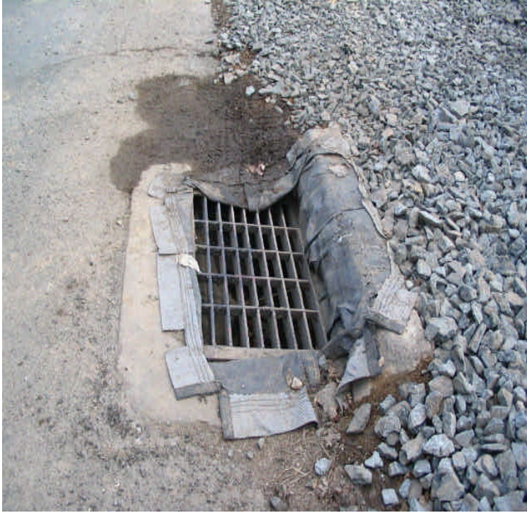
View of the catch basin located immediately adjacent to the access off Sunset Drive. The silt sack was pulled over the curb drop inlet here to provide further protection.
