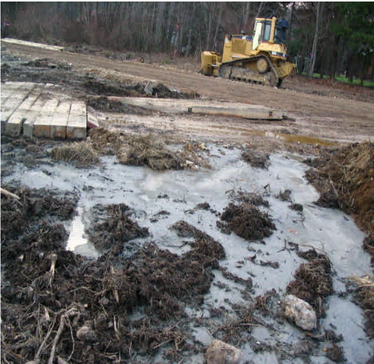
An additional view of the sediment/slurry flowing toward the wetland off Sunset Drive.
