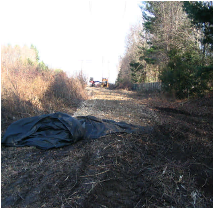
View of the catch basin located immediately adjacent to the access off Sunset Drive. The silt sack was pulled over the curb drop inlet here to provide further protection.
