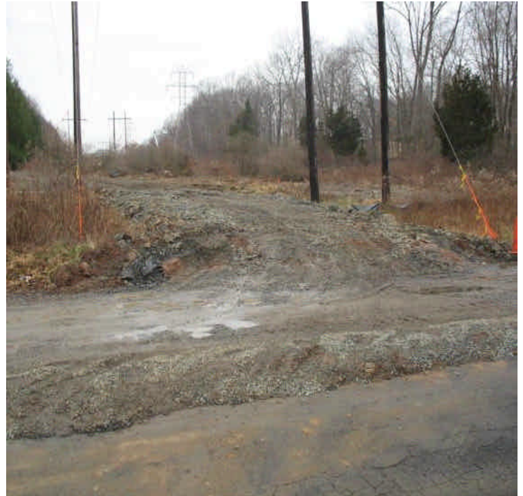
Continue to monitor run-off seeping from non-federally jurisdictional wetland crossing off Old Farm Rd.
