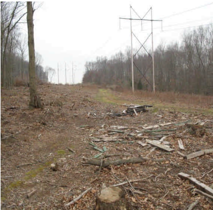
ROW off Stony Brook Rd. Non-project related debris has been dumped in this area.
