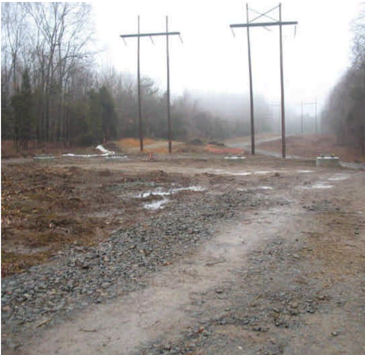
ROW access road and foundations in place off Black Walnut Dr.
