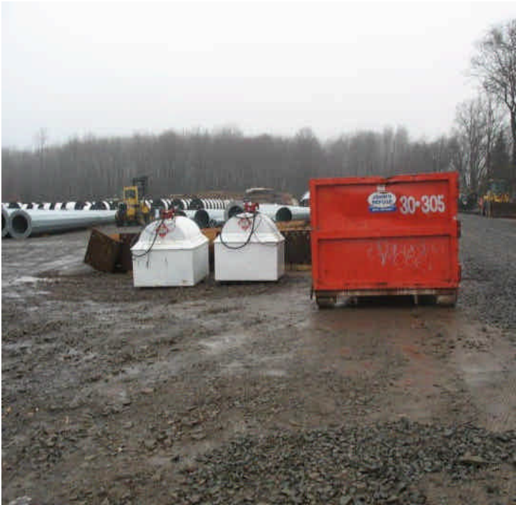
Fuel tanks and dumpster were moved farther from the wetland; controls for the fuel tank nozzles should be reinstalled.
