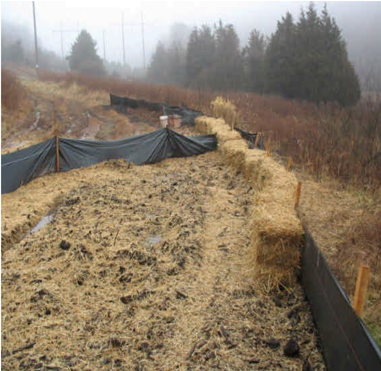
Slurry was pulled back from the edge of the silt fence at Black Pond and new haybales were installed. Mulch has been spread around the site for increased, temporary stabilization.
