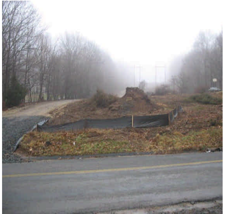
Silt fence, clearing, grading, and access road off Arbutus Street. Pull back stone from the roadway as needed.
