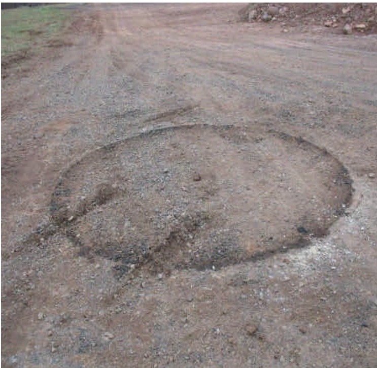
A stain was noted along the access road to the ROW north of Beseck SS. It is unclear whether this resulted from material storage or an equipment leak. Regardless, the size is non-reportable.
