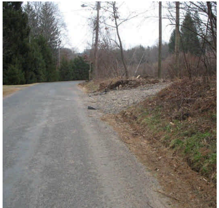
ROW entrance off Little Lane. No sediment tracking was noted.
