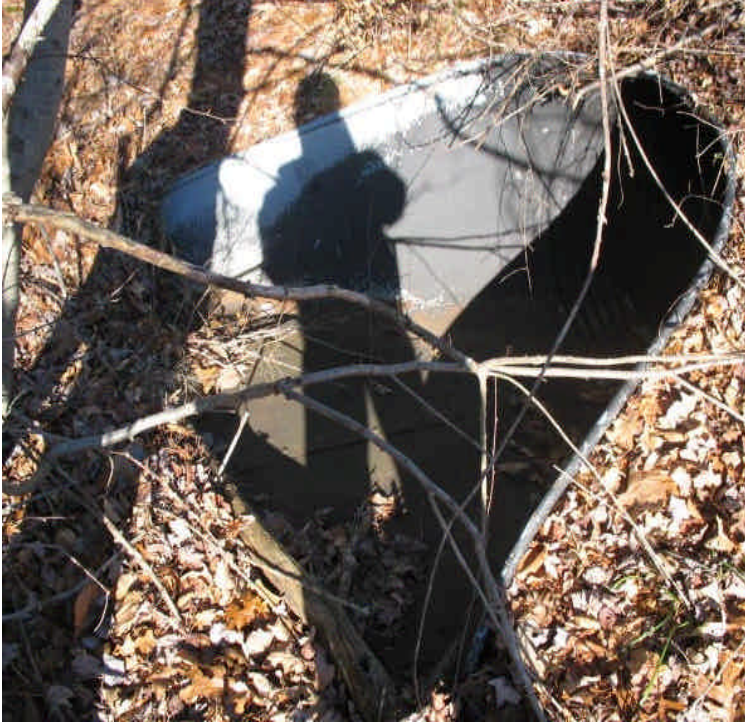
View of the culvert under the access drive. No sediment issues have been observed.
