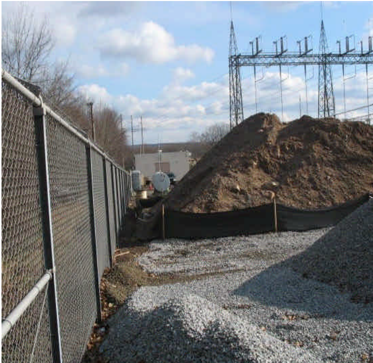
The remaining soil stockpile is surrounded by silt fence. Remove soil from site when feasible.
