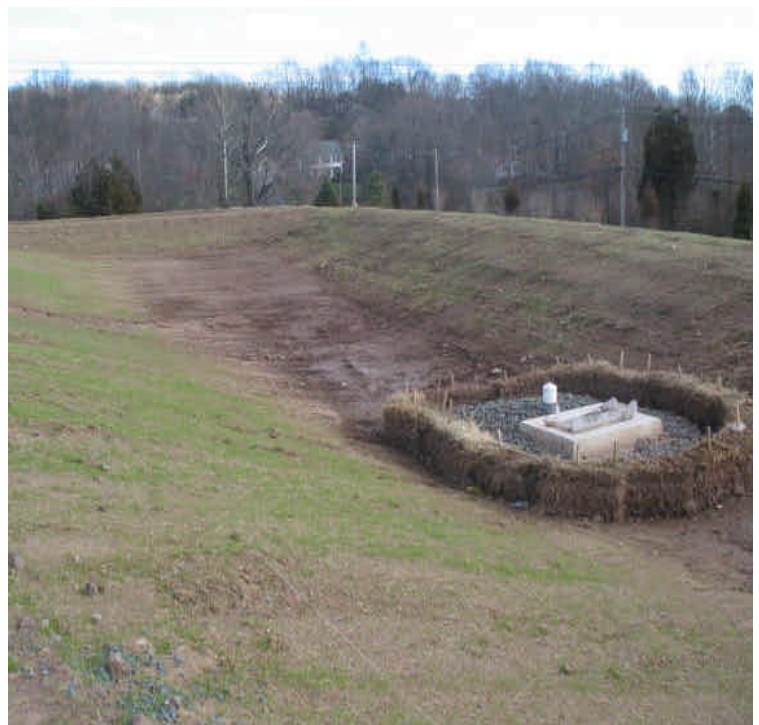
Some grass cover was observed on the seeded slopes of the detention basins. Additional/alternative controls are still recommended to prevent turbid water from reaching the inlet.
