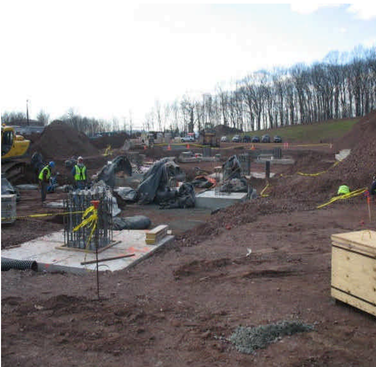
View of site looking from east to west. Foundation installation continues.
