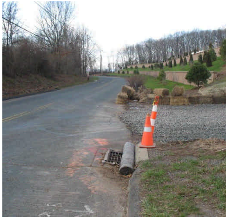
View of Carpenter Lane and retaining walls. No sediment was noted leaving the site entrance. Minor sediment was noted in the gutters.
