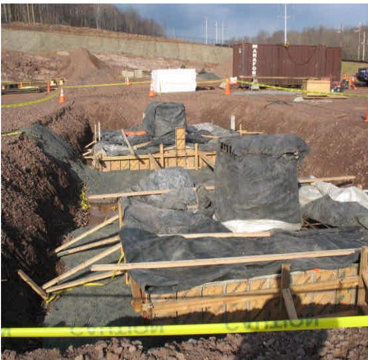
View of site looking from south to north. Foundation installation continues.
