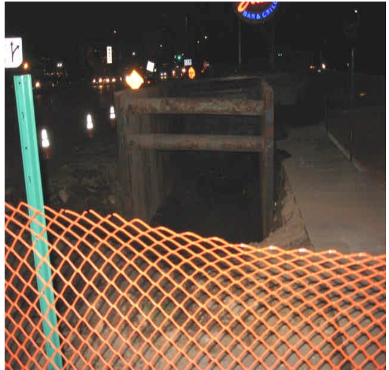
Vault #7536 construction. Four ornamental plum trees were removed for vault construction.
