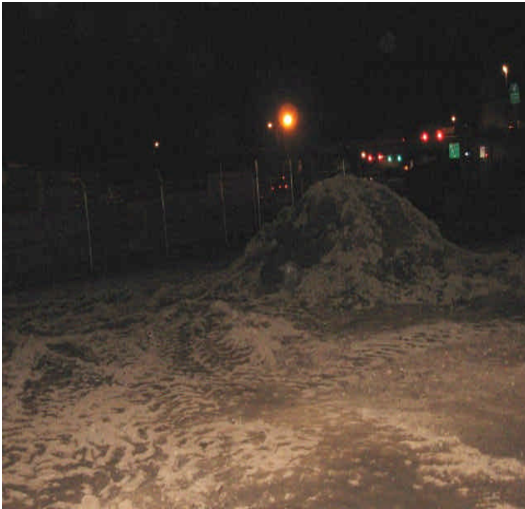
Photograph of soil pile at the intersection of Railroad Ave. and Wordin Ave. If pile is to remain, it should be temporarily stabilized.
