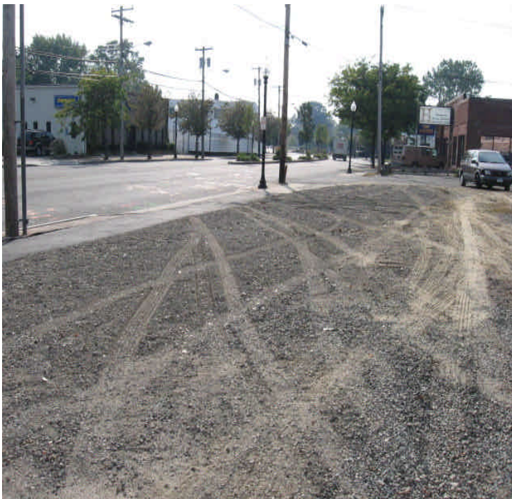
Location of Vault # 7539 which was installed last week.
