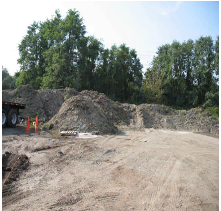
Inactive soil piles within the yard. If the resulting soil piles have been or will be inactive for 30 days they should be seeded appropriately to control dust production.
