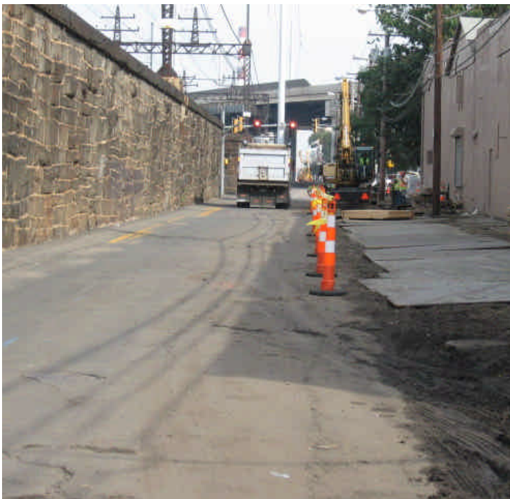
Trenching work on Railroad Ave. between Iranistan Ave. and Howard Ave.
