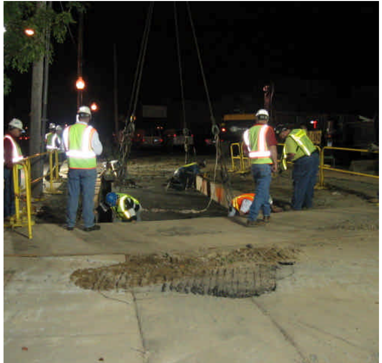
Photo of Vault #7439 in Bridgeport being lowered into the trench.
