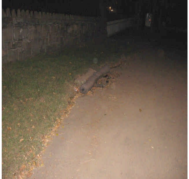
Catch basin properly protected in Old Post Rd. The inlet receives stormwater runoff from activities in front of the Fairfield Inn.
