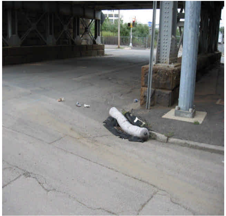
Catch basin protected at the intersection of Railroad Ave. and Hancock Ave.
