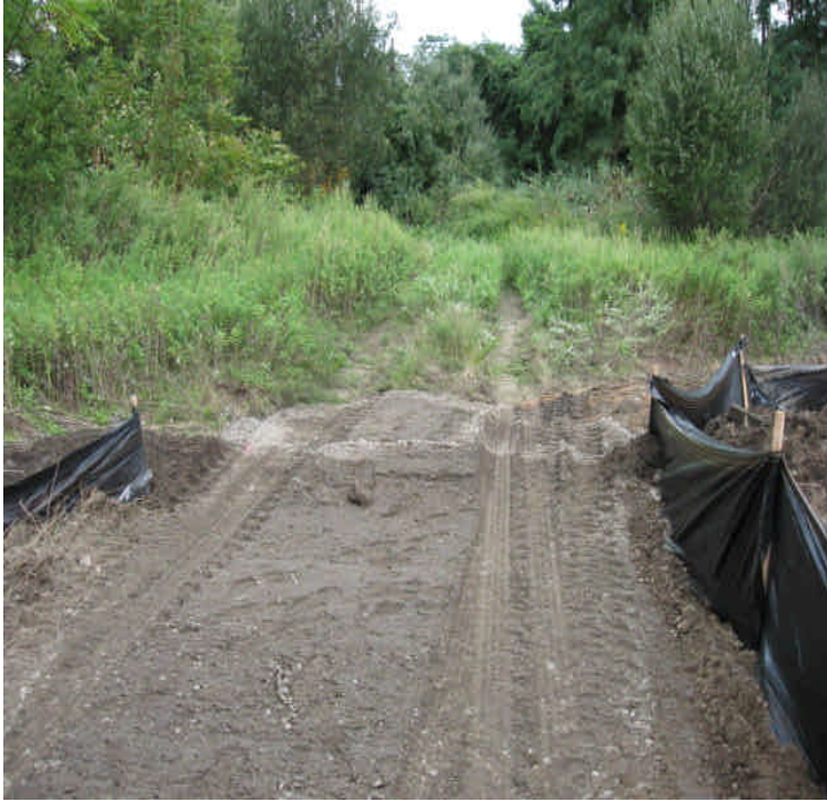
Photograph of area within the Kings Highway storage yard that requires regular access by the Fairfield Sewer Dept. The access way can not be closed off with silt fence, other methods of control will be implemented. (i.e. stone berms)
