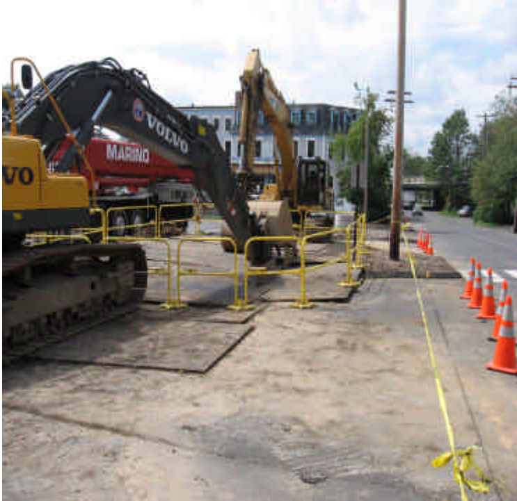
Photograph of vault #6428 construction on Old Post Road. It appears that sweeping the sediment from the asphalt had been attempted, but some was left behind. Watch for sediment migration or dust production and re-sweep if necessary.
