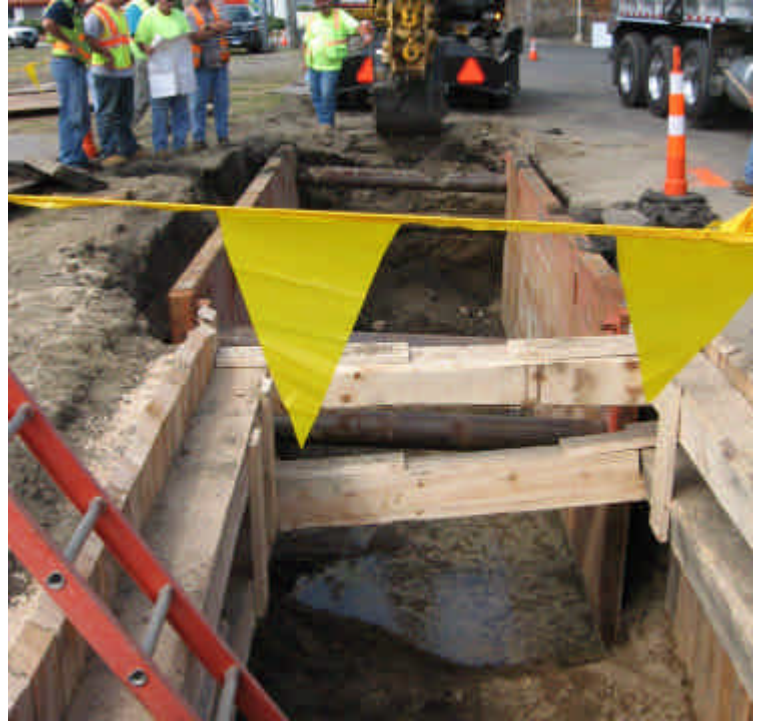
Photo of trench and associated shoring being prepared for conduit installation.
